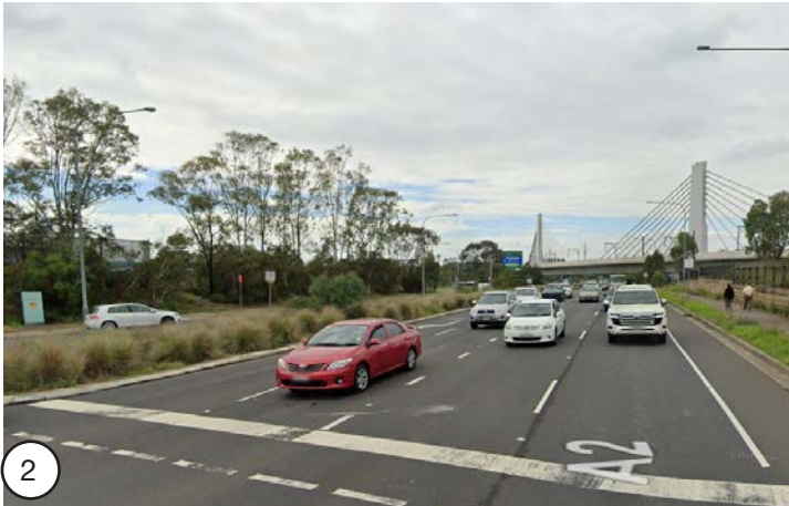
2 Windsor Road is a key arterial route. Existing canopy trees between the hospital site and road are proposed for retention.
