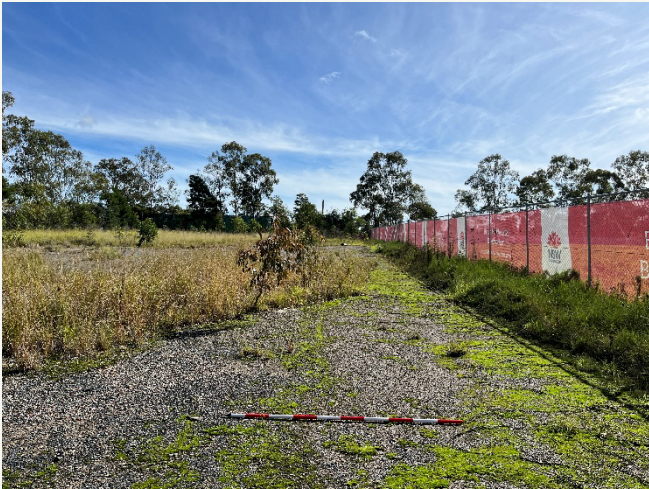
Plate 7: Moss and grass have begun to grow over the asphalt/ gravel hardstand area; facing north
