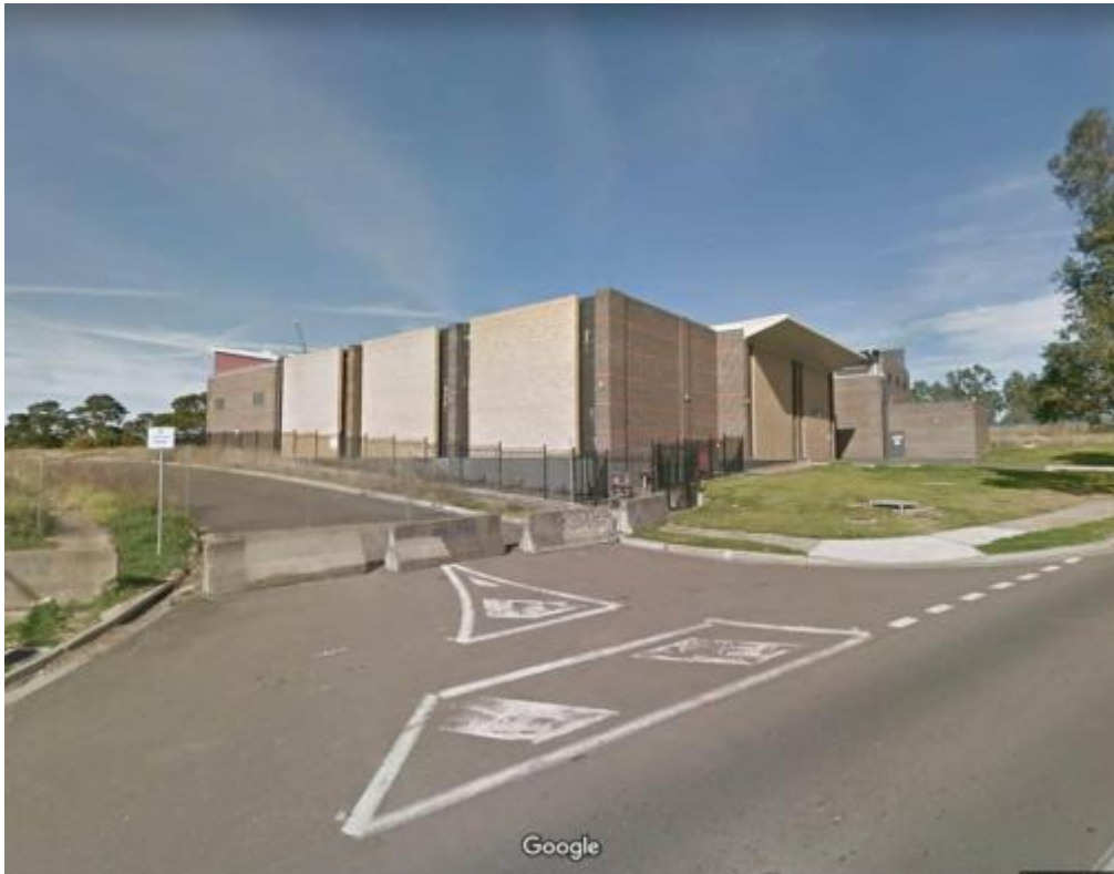
Figure 8: Mungerie Park Zone Substation transformer runway
