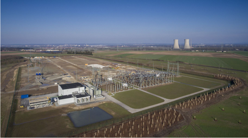
Figure 2: Example of Synchronous Condenser
