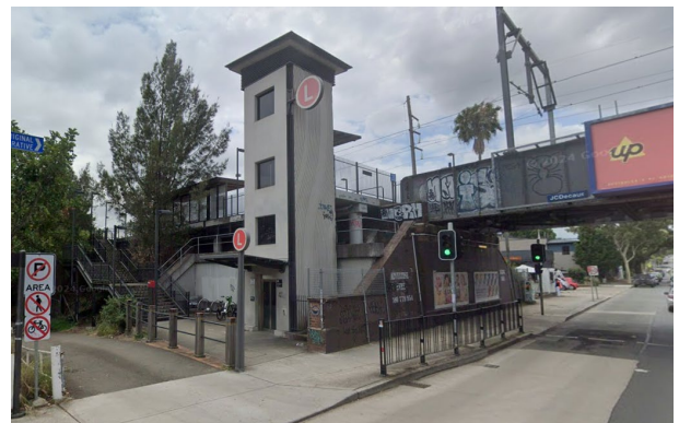
Figure 8 View of light rail stop to the west of the site
