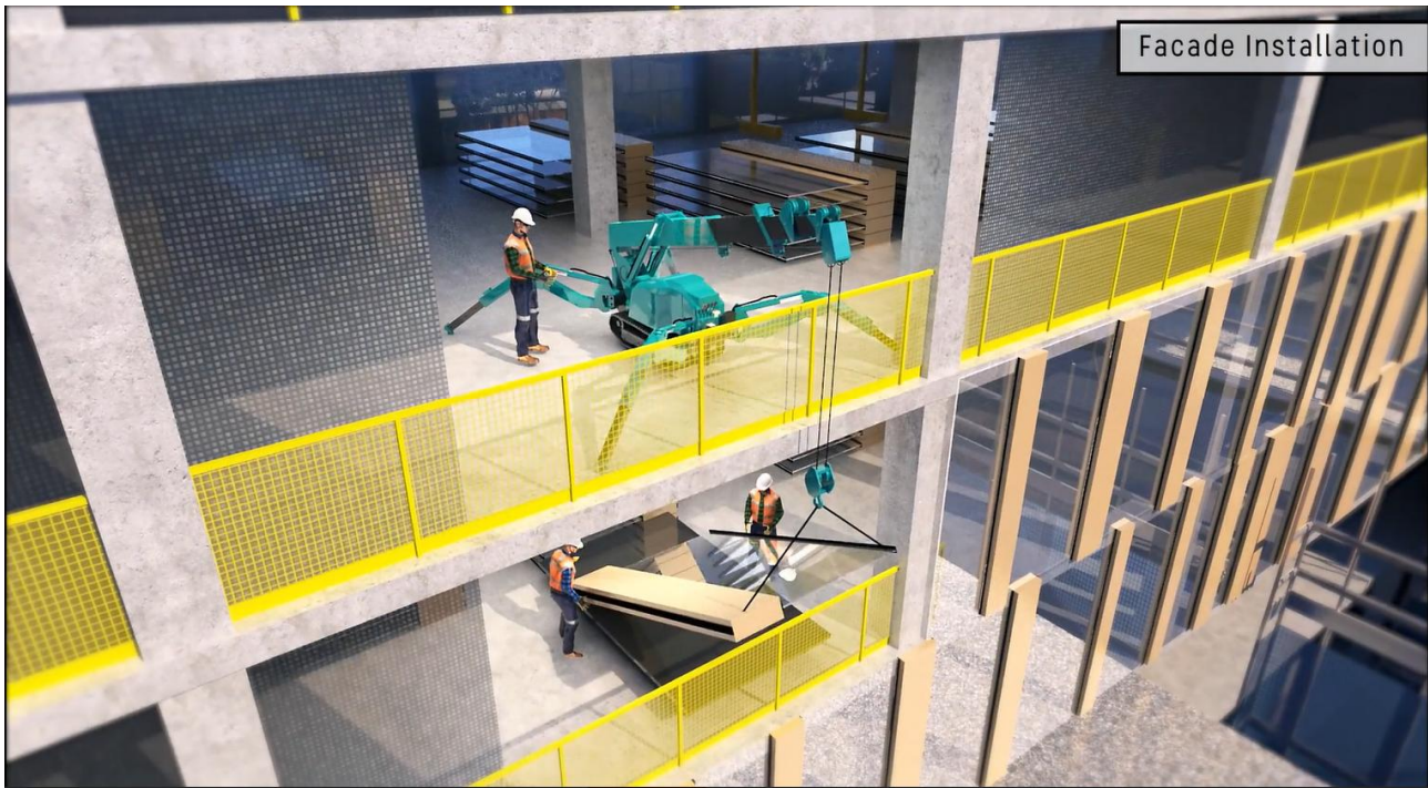
Figure 10 Curtain Wall Façade Installation methodology
