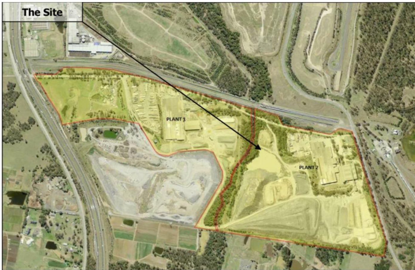
Figure 1 The Site – Aerial View (SIXMaps, 2018)
