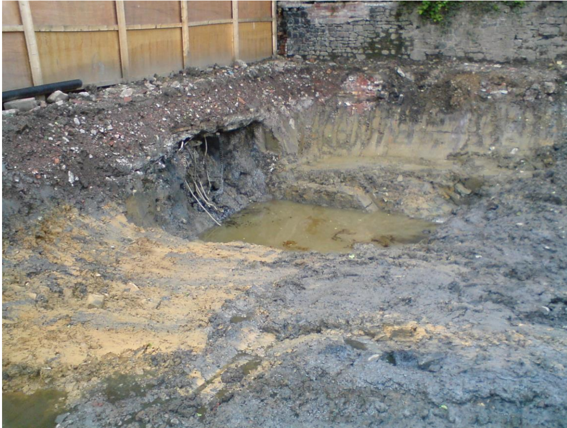
Figure A1 – Differing colours and texture of soil may indicate contamination
