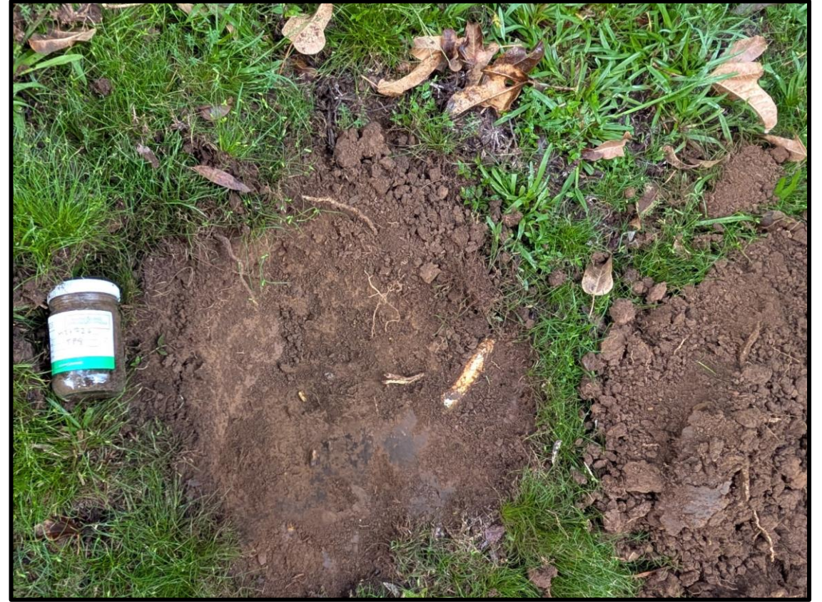
Figure 17. TP8 test pit excavation.
