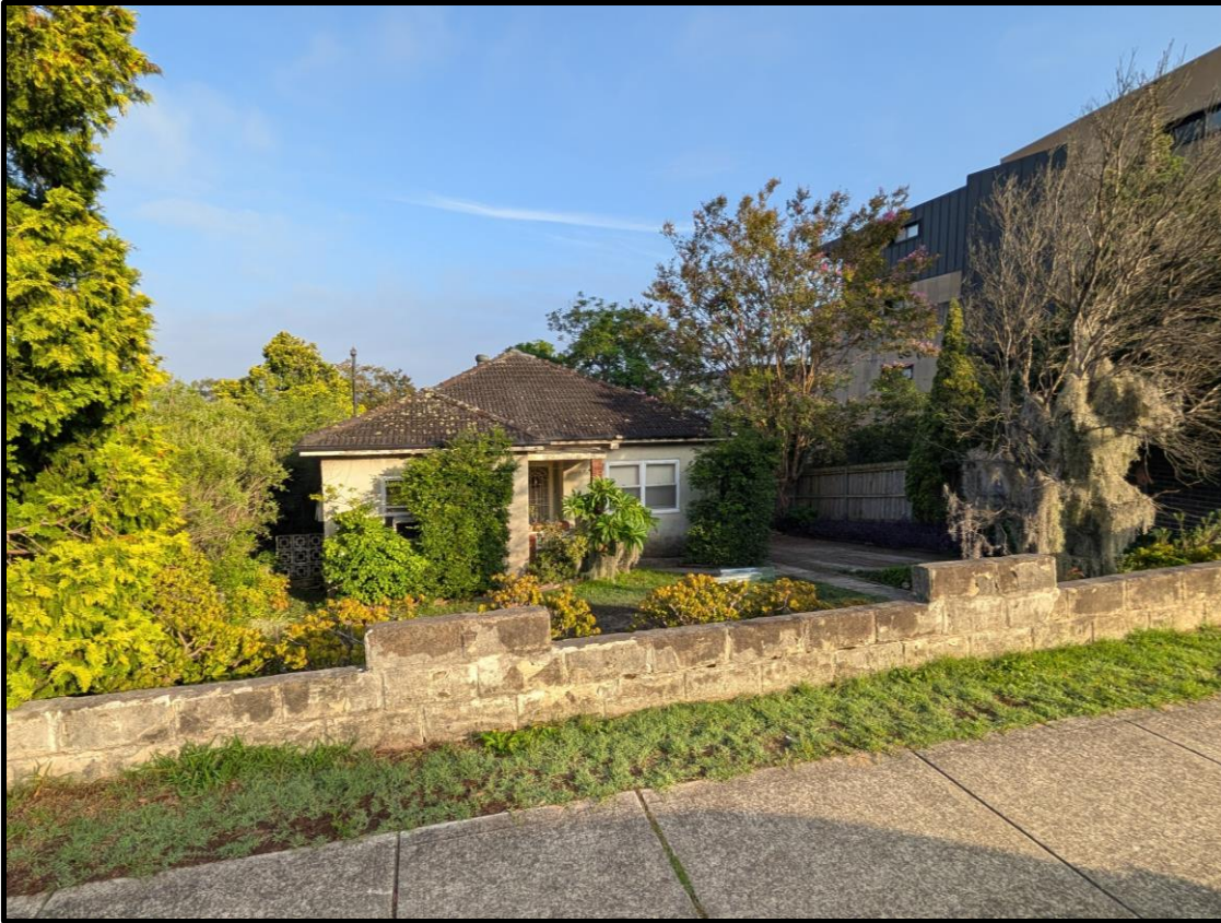
Figure 14. Front view No. 174.
