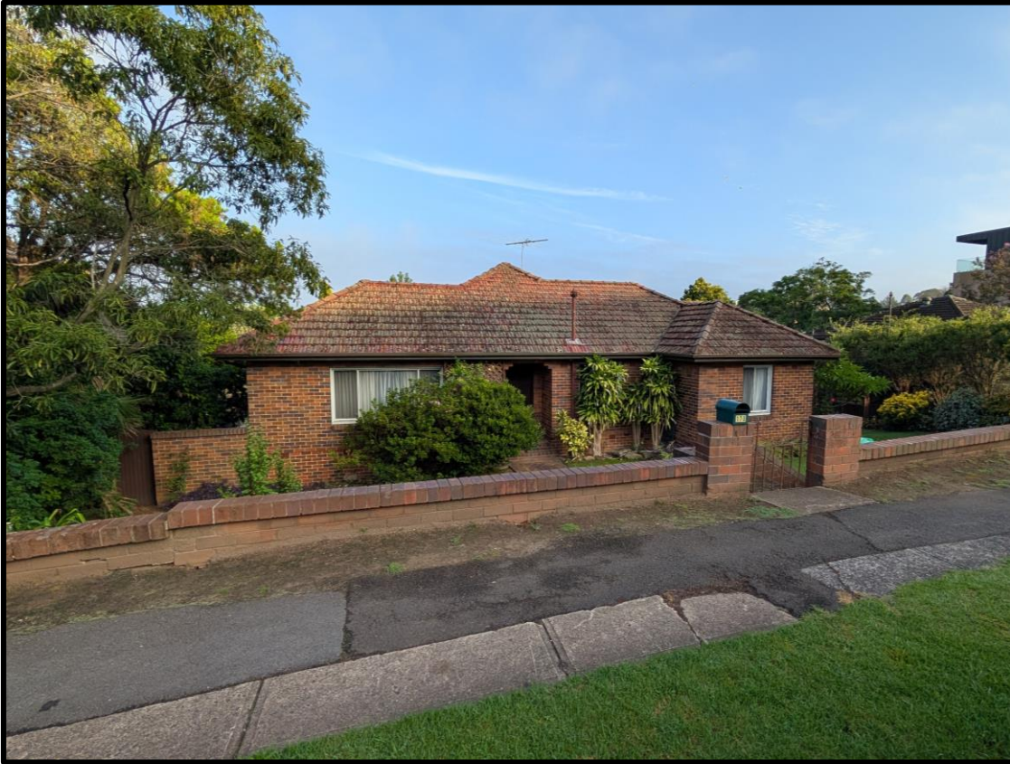
Figure 12. Front view No. 170-172.
