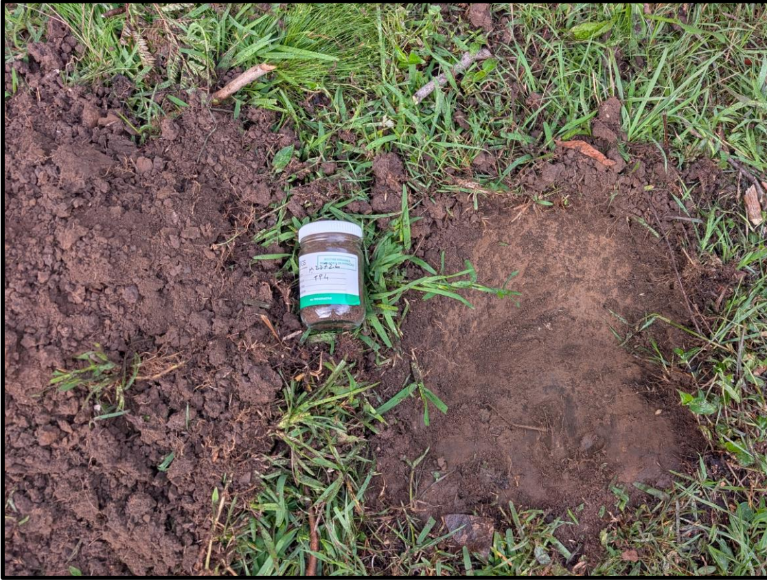
Figure 16. TP41 test pit excavation.
