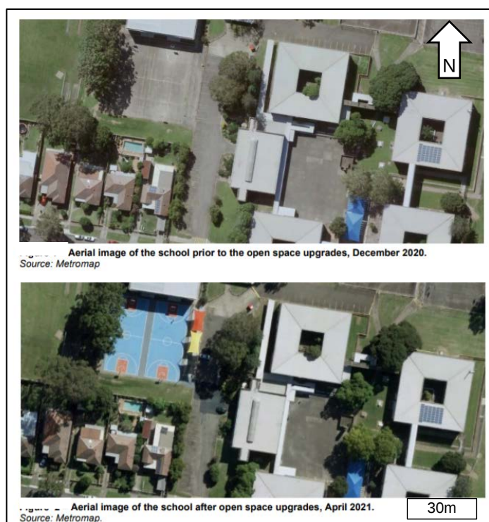
Figure 28 | Aerial photo of recent upgrade works (Source: Applicant's supplementary information 2021)
