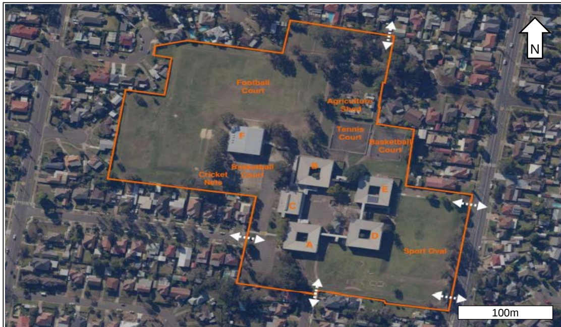
Figure 3 | Aerial view of existing building and structures on-site (Source: Applicant's EIS 2021)
