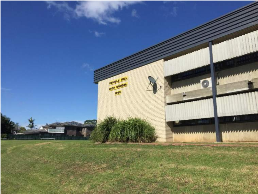
Photo 3: Photo of existing building.
