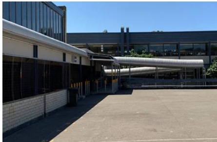
Figure 11 Internal view of playground
