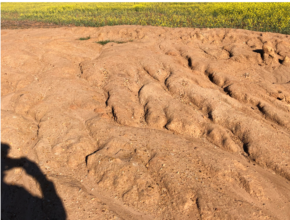
Photo 8.6. Farm dam earthen embankment showing erosion channels
