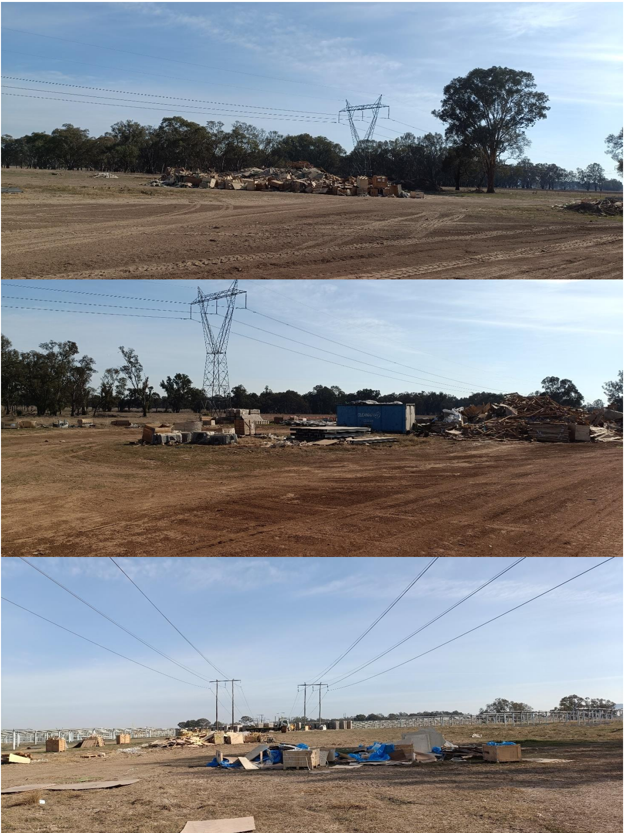
Photograph C.3 Waste material storage – materials not separated and numerous sites of this nature across site at the time of the audit.
