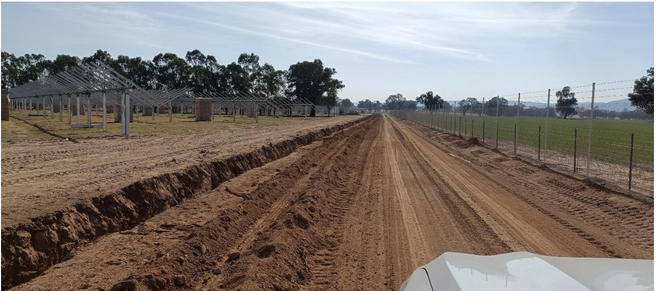
Photograph 3.2 Trenching works for cabling installation commencement
