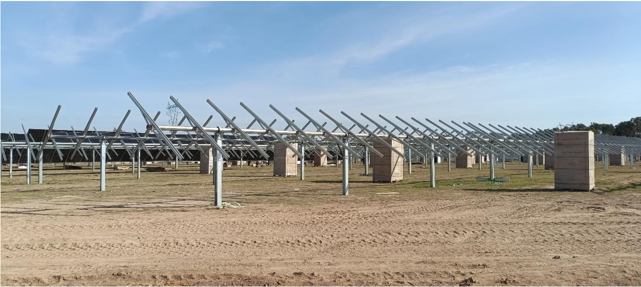
Photograph C.2 Arrays ready for panel installation
