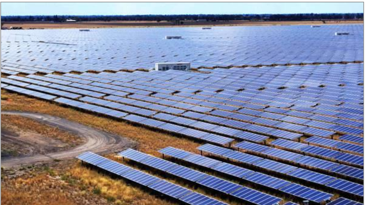
Figure A-2: Fully assembled tracking array solar farm showing inverter housing (image courtesy Nextracker Australia, actual tracking system may differ)
