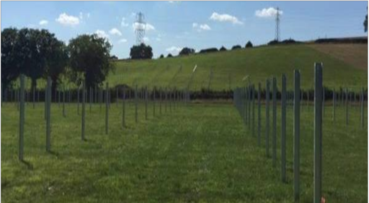
Figure A-1: Piles for the solar farm in place (image source Infinergy UK)
