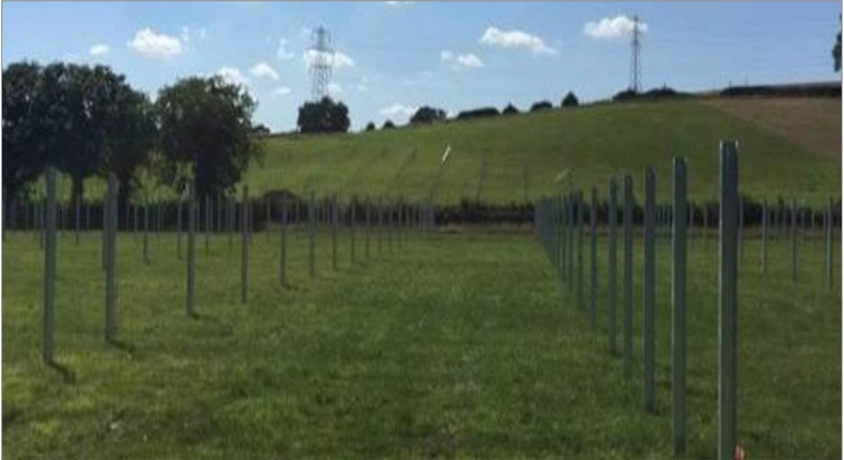
Figure 4-3: Piles for the solar farm in place (image source Infinergy UK)
