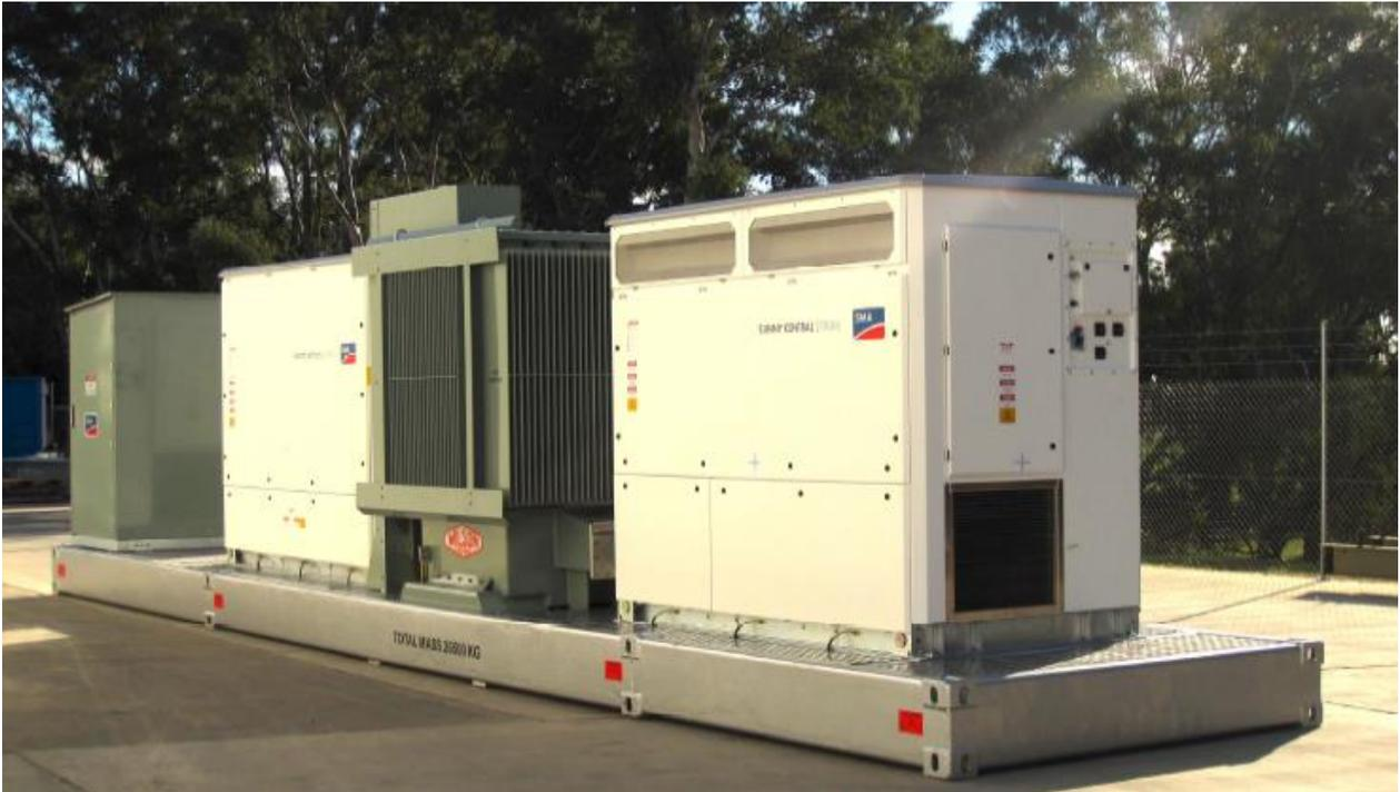
Figure 4-7: SMA MVPS Skid Mounted Solution (image courtesy of SMA)
