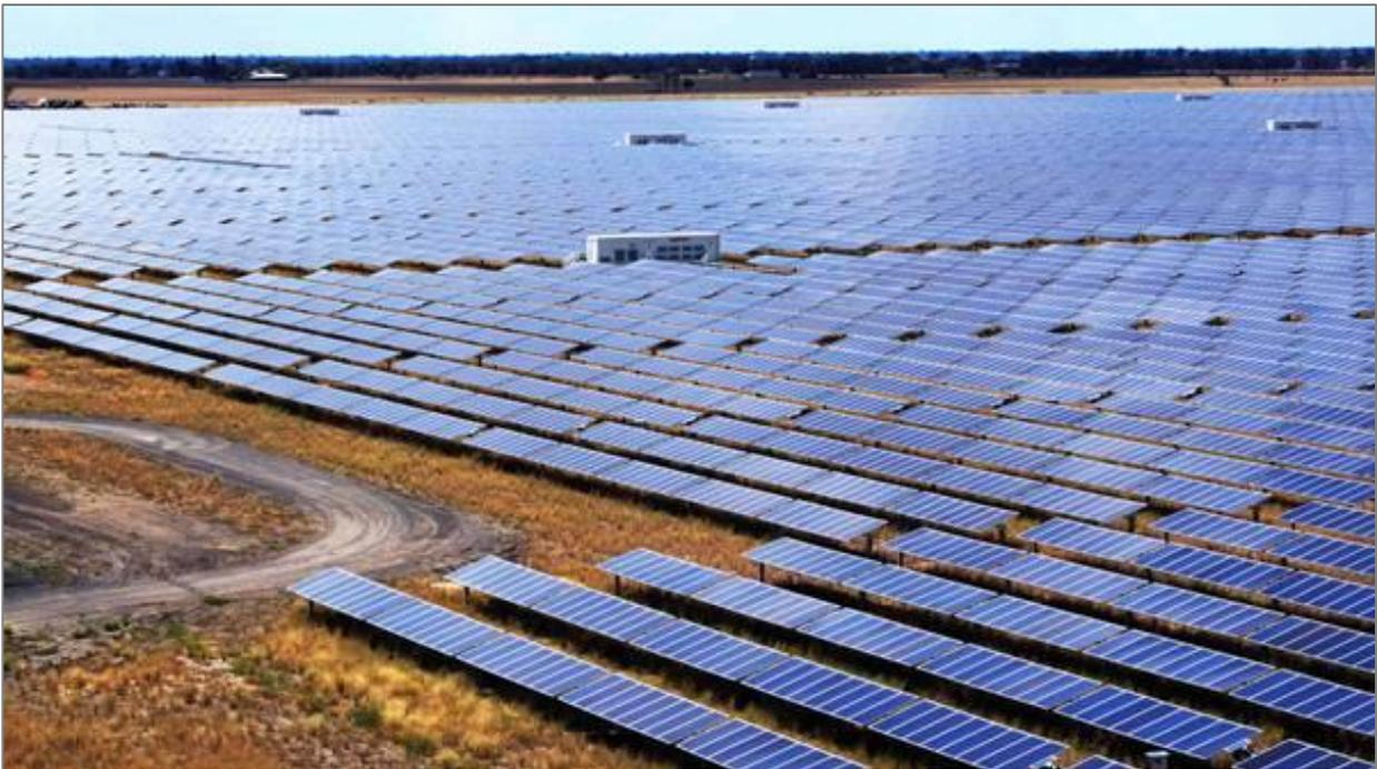
Figure 4-4: Fully assembled tracking array solar farm showing inverter housing (image courtesy Nexttracker Australia, actual tracking system may differ)
