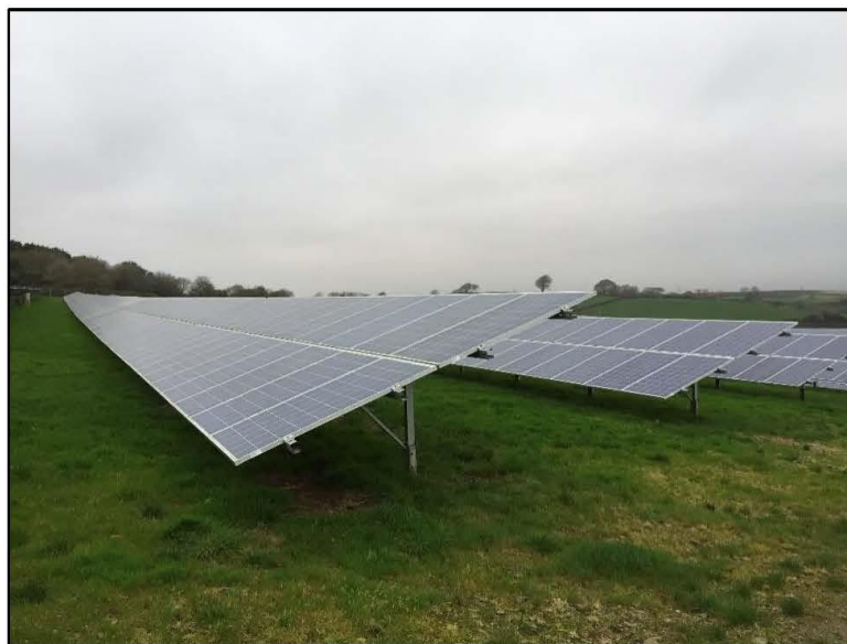
Figure 2: Typical height of a Solar Farm panel and general arrangement
