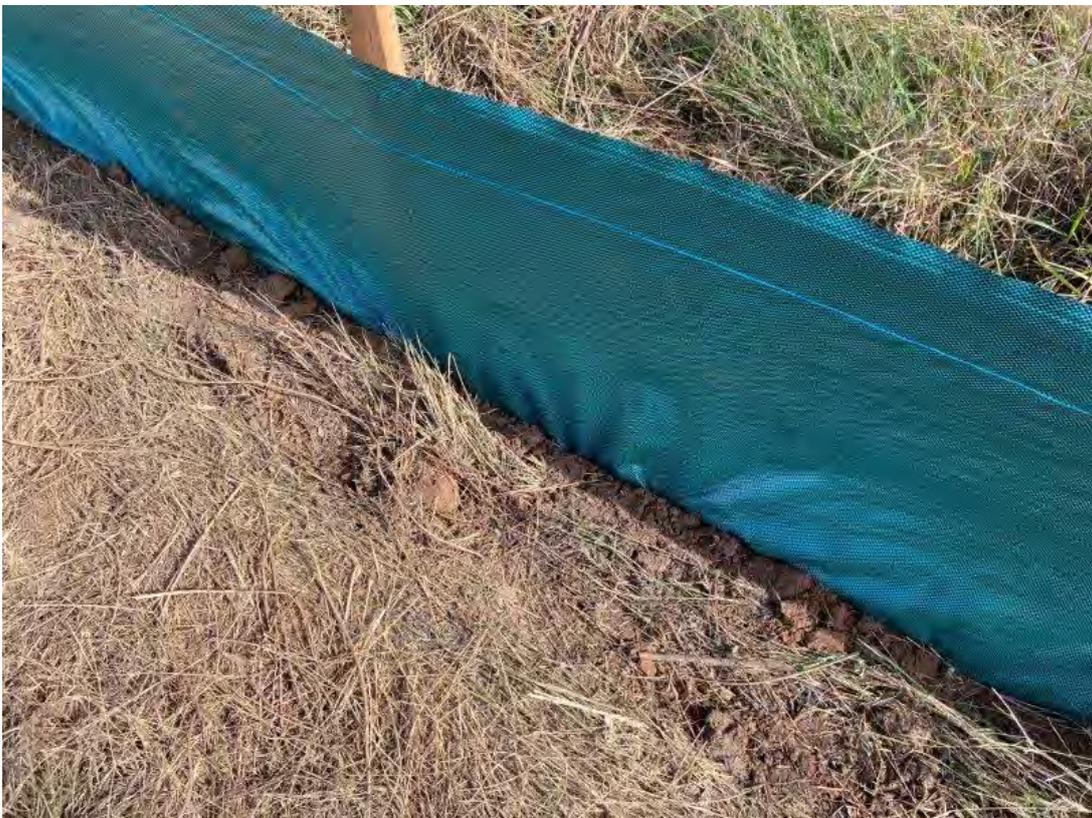
Plate 36 – Sediment fence installed to temporary access track prior to permanent road construction
