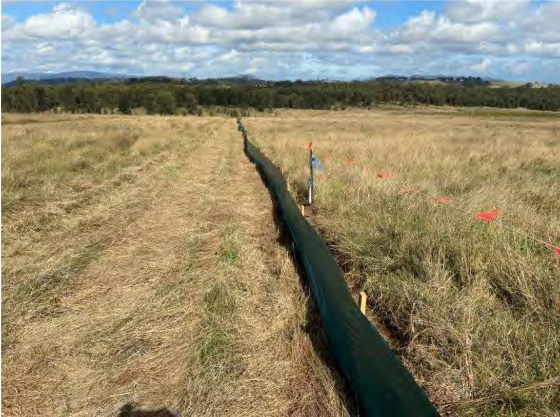
Plate 35 – Sediment fence installed to temporary access track prior to permanent road construction
