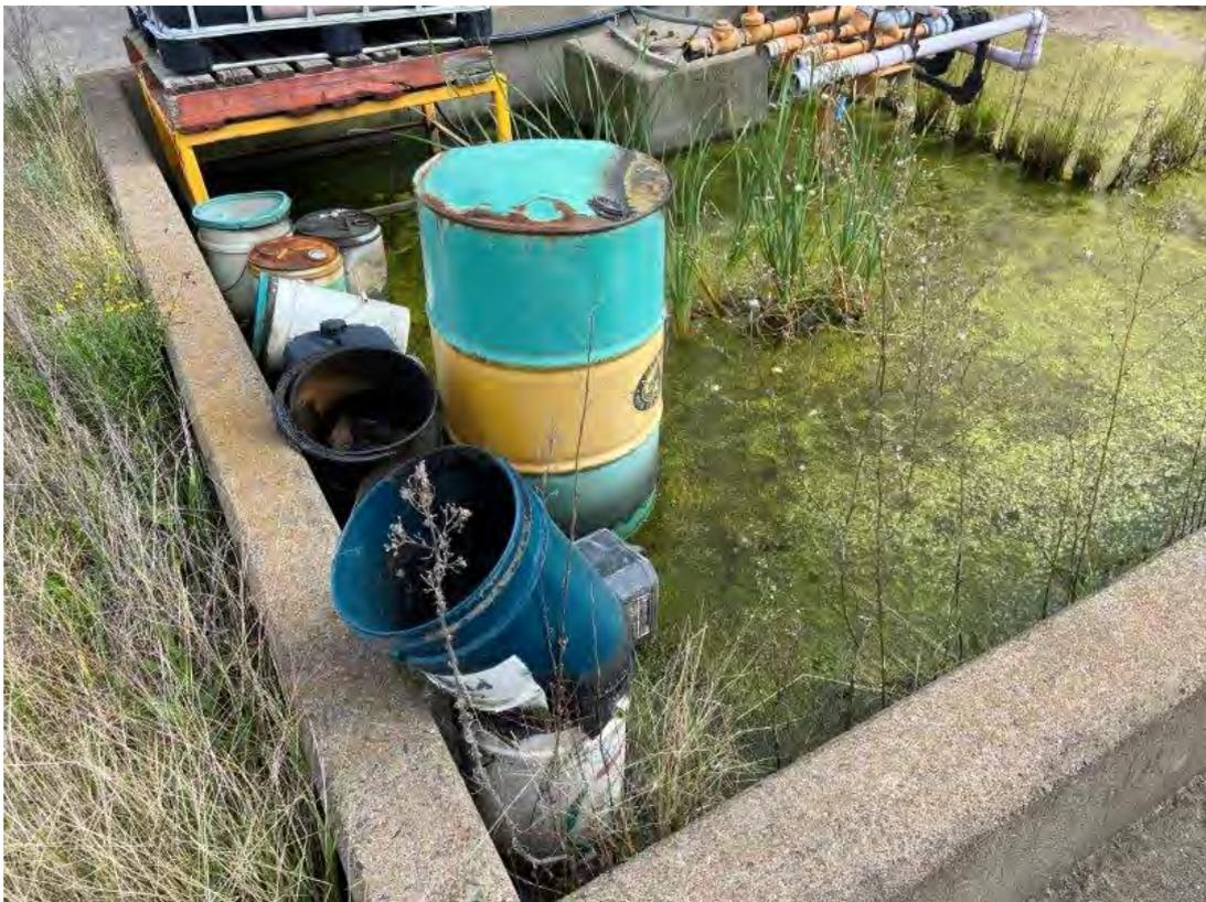
Plate 22 – Bund requiring clean out and with open containers present
