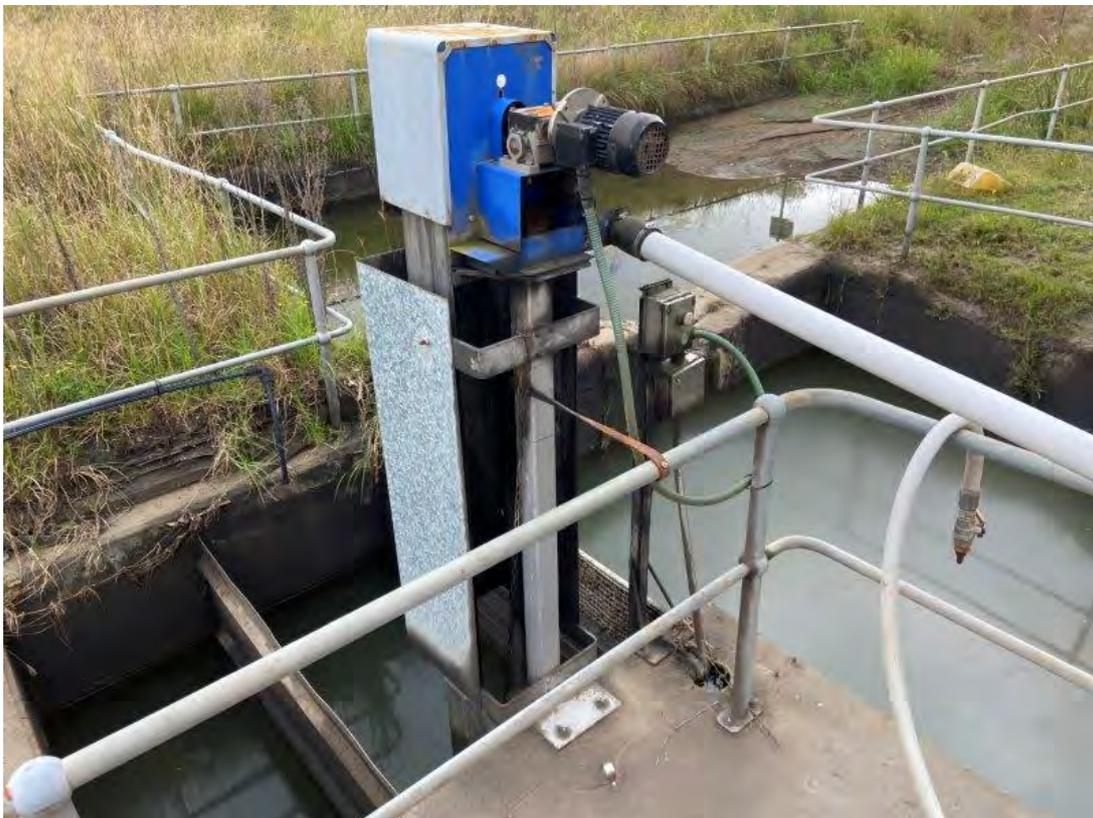
Plate 20 – Oily water separator off workshop area
