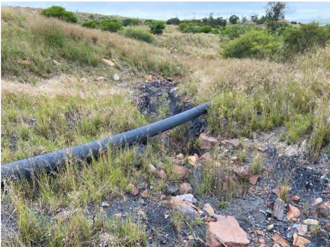
Plate 48 – Evidence of gully erosion through dirty water drainage channel to southern void
