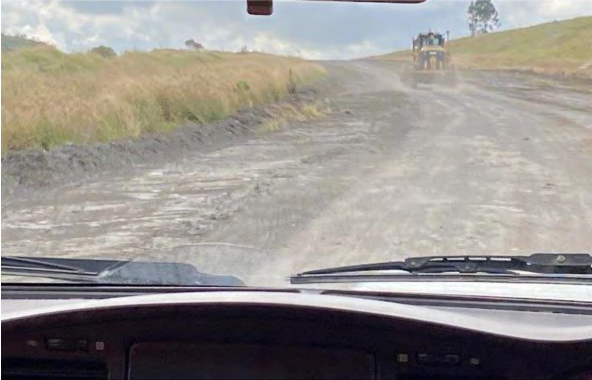
Plate 39 – Wheel generated dust from mobile plant on haul road
