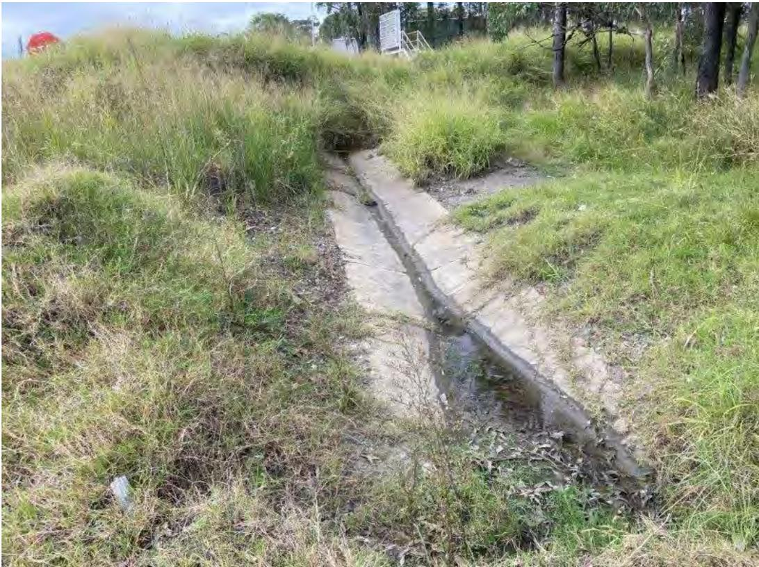
Plate 18 – Concrete swale drains overgrown near workshop
