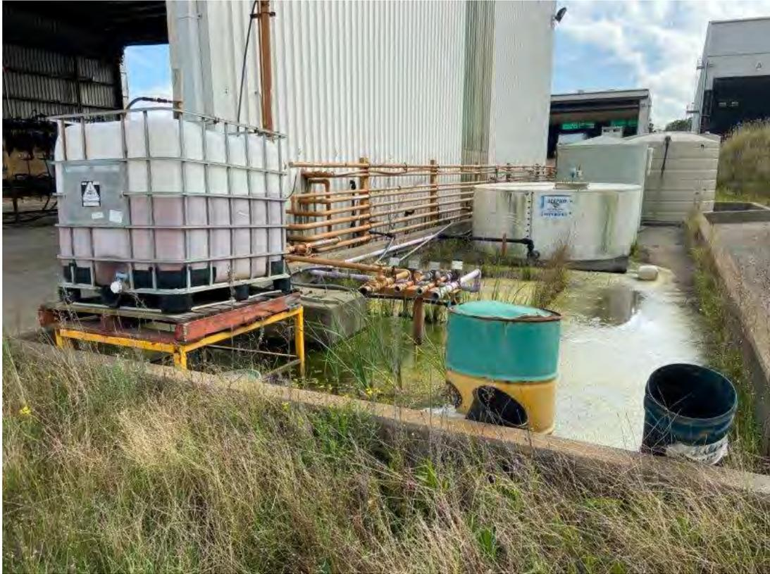
Plate 21 – Bund requiring clean out and with open containers present
