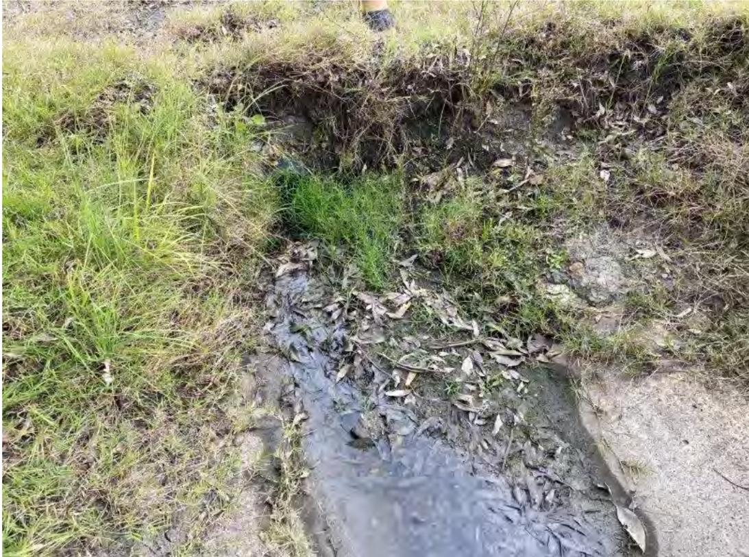
Plate 19 – Under road pipe blocked leading from wash bay to oily water separator
