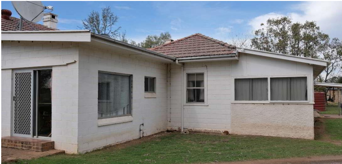
Figure 31 – View of the south-east corner of Bowfield, showing the hip roof of the second wing constructed in off form concrete with an embossed block pattern and timber sash window dating to the c.1950s. The skillion roofed wing at the left is part of the c.1960s front wing of the homestead.
