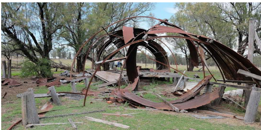
Figure 36 – View of the collapsed rear (southern end) of the Nissen Hut with only the perimeter posts remaining in their original location. The flooring is completely missing with only a small area of collapsed roofing existing.
