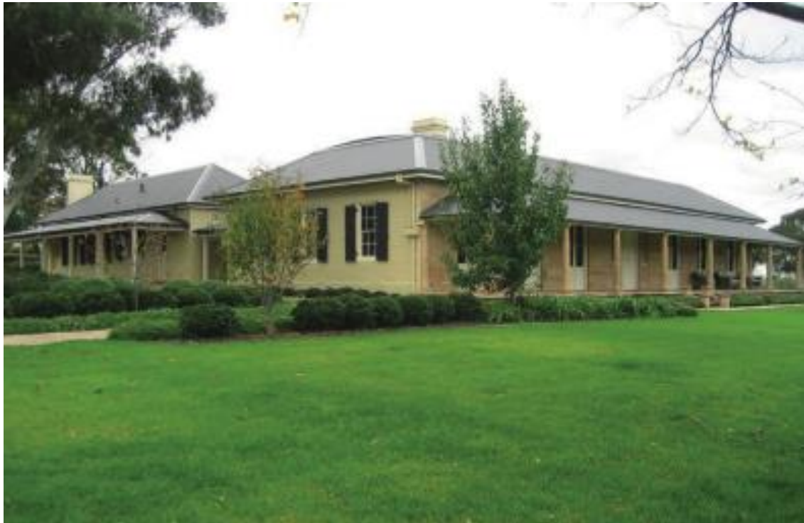
Figure 42 – View of Woodlands Homestead M07 (Source: AECOM 2015).
