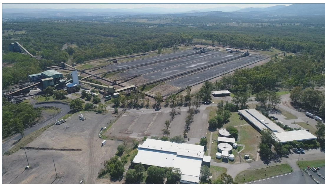
Plate 1-1 – Existing Maxwell Infrastructure
