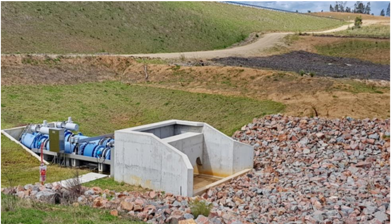
Photo 22 Typical Engineered Pipeline Outfall Stilling Basin
