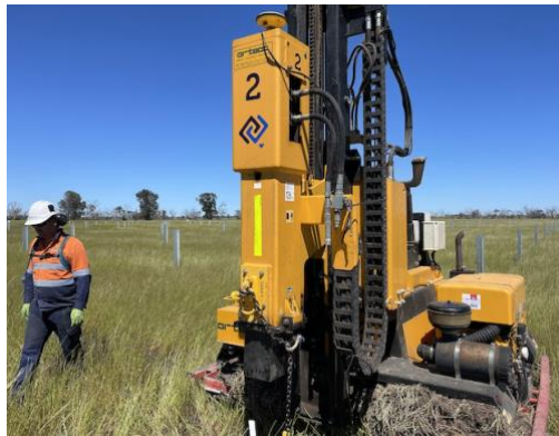
Photo 10: Piling rig on site.
