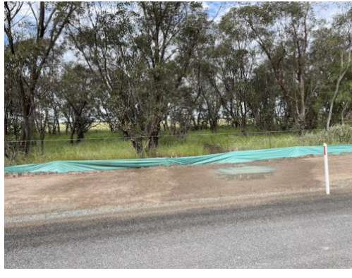
Photo 20: Sediment fencing at discharge location adjacent site access way and Gordon's Lane.
