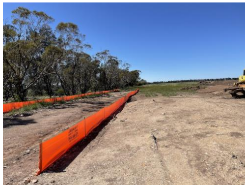
Photo 4: Sediment fencing install on down-slope perimeter, adjacent Gordons Lane.
