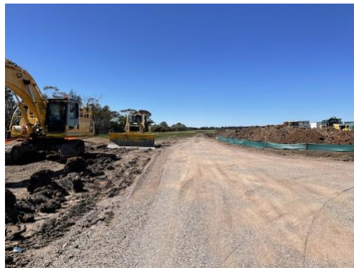
Photo 3: Internal access tracks being constructed. Not yet constructed as all-weather access. Stockpile protected with sediment fencing.
