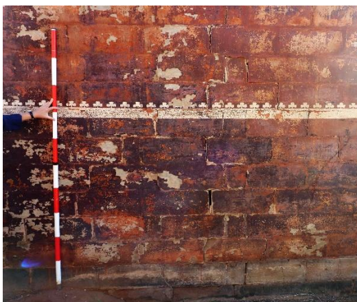
Figure 29: Wash paint and decal to interior wall of common room
