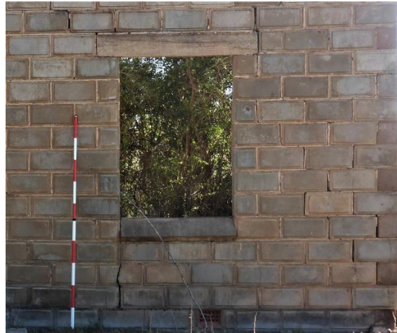
Figure 28: Concrete blocks showing surface finish and window treatment. Exterior view
