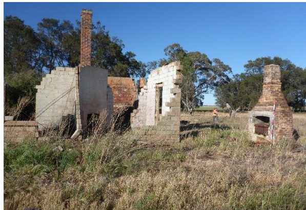
Figure 24: Structure in Lot 18 showing brick chimneys. View west
