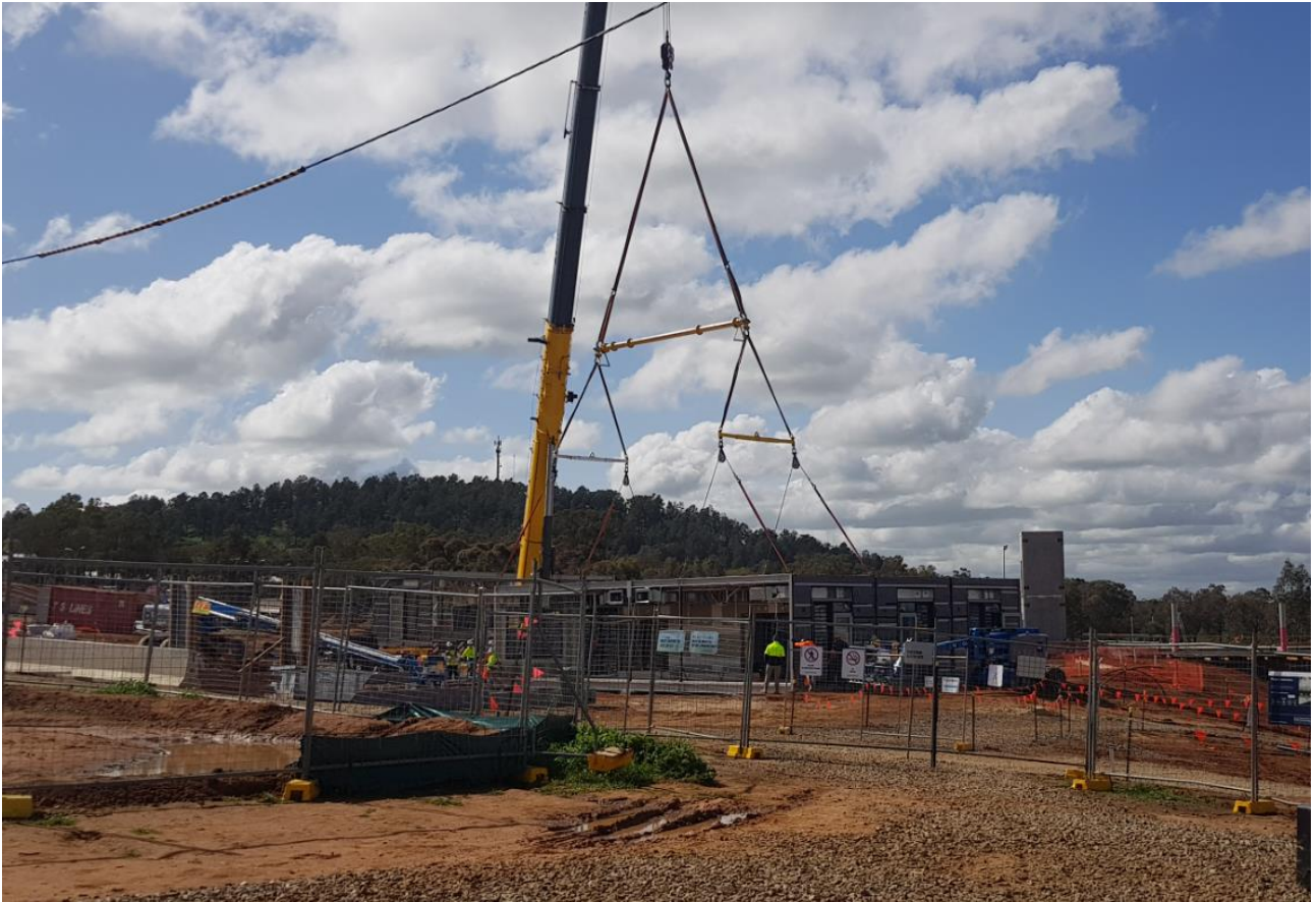
Photo 11: Lifting of modular section of building.
