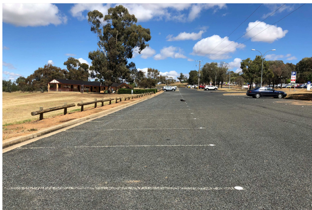
Figure 16 Northern CSU car park CP04
