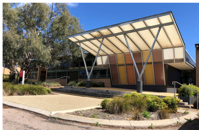
Figure 19 CSU campus Building 21
