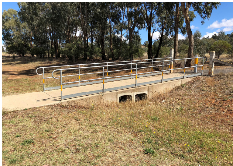
Figure 15 Existing stormwater channel adjacent to Estella Road
