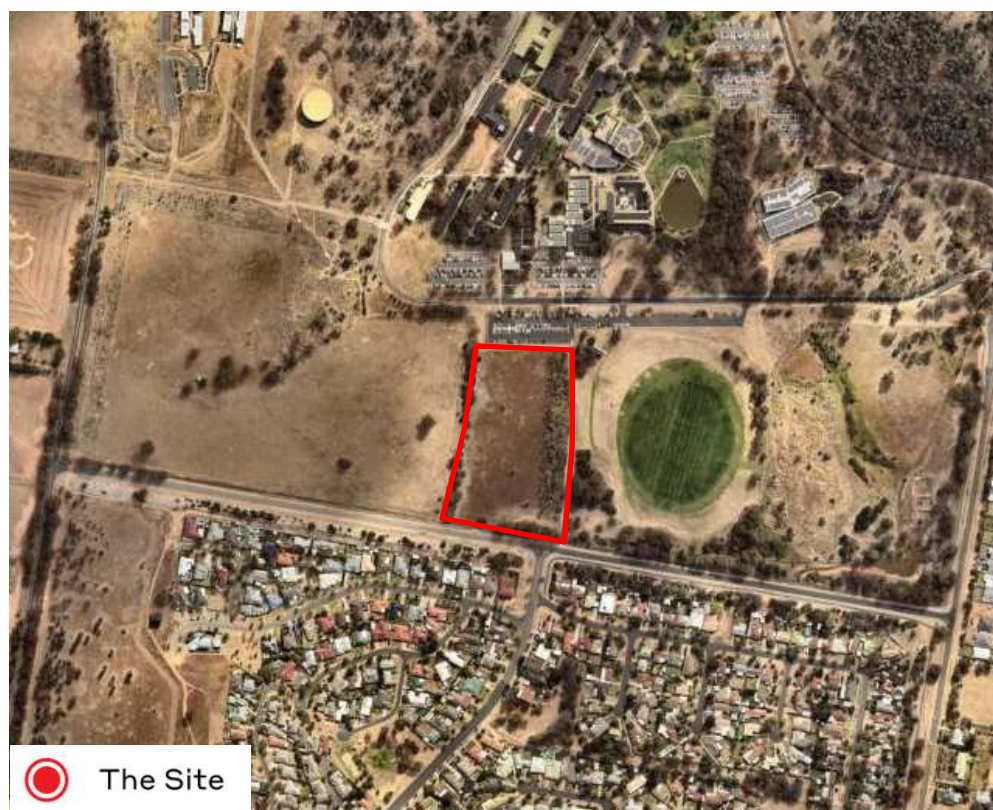
Figure 2 Aerial photograph of site and surrounds
