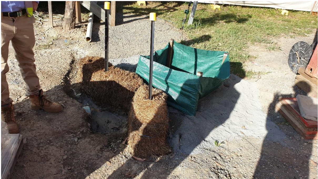
Plate 4 – Straw bale and silt fence at outlet from rock lined settling basin
