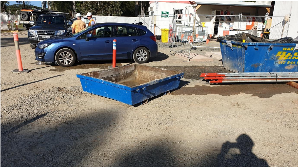
Plate 2 – Concrete washout tray
