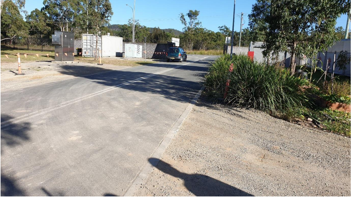
Plate 1 – Clean access road to site
