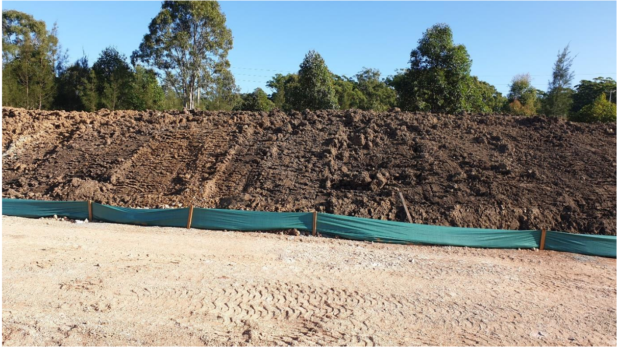
Plate 3 – Silt fence at base of topsoil stockpile
