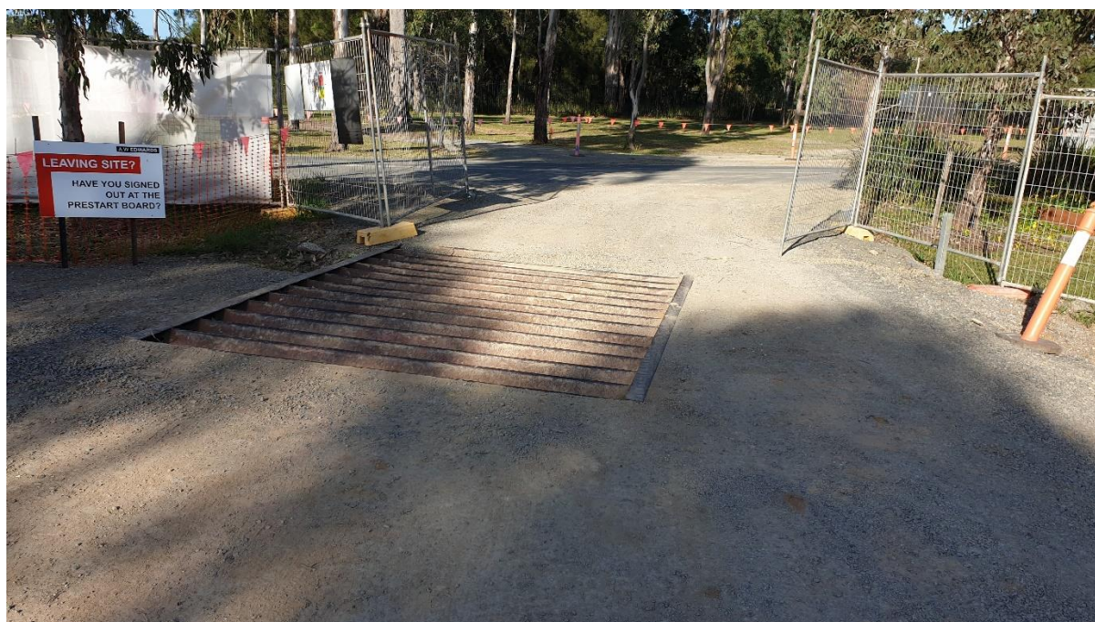
Plate 9– Wheel shaker installed at exit from site
