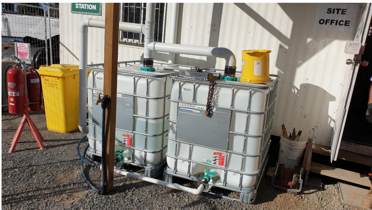
Plate 8 – Rainwater collection tanks for reuse on site
