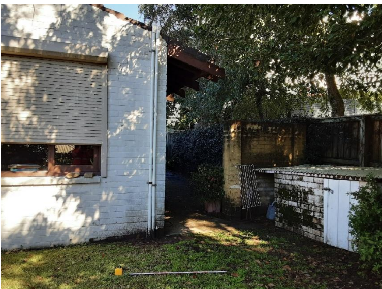
Photo 17 Example of residential development and utilities at 6 Ku-ring-gai Road in the central portion of the study area, facing south
