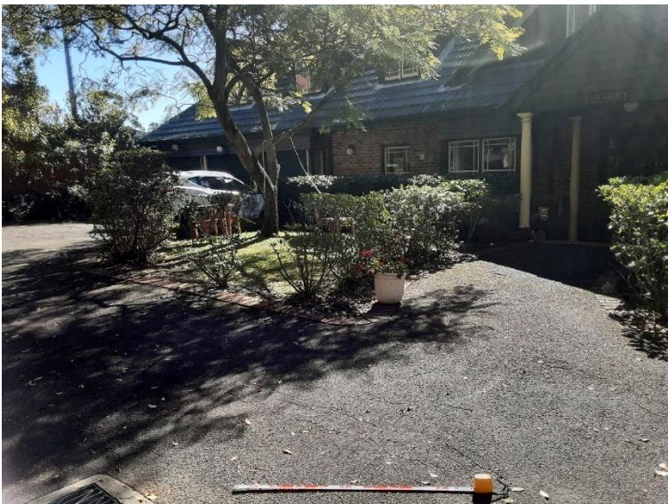
Photo 19 Example of residential development and subsurface drainage at 5 Nulla Nulla Drive in the central portion of the study area, facing south
