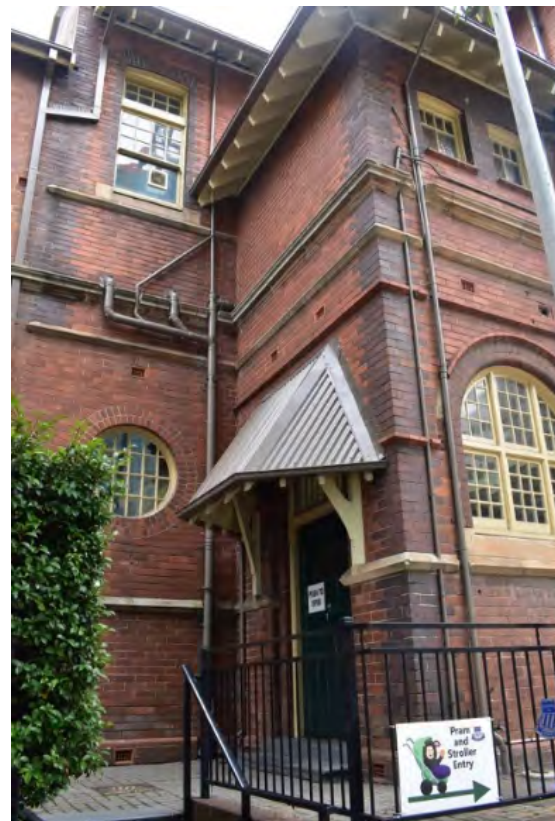
Figure 16 Photograph taken at the public entry point to the school, looking towards the 1902/03 phase of construction (lower portion) and the 1915 phase of construction (upper portion). Note the seamless integration of the two. Source: May Willard, 11 th January 2018.
