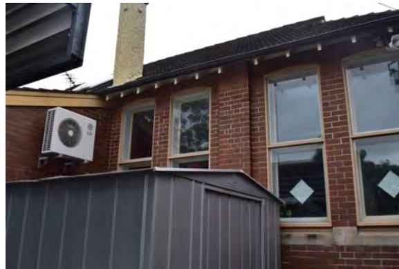
Figure 20 Photograph taken from directly in front of the 1908 extension, with sandstone copings to windowsills and rough cast chimney. Source: May Willard 11 th January 2018.
