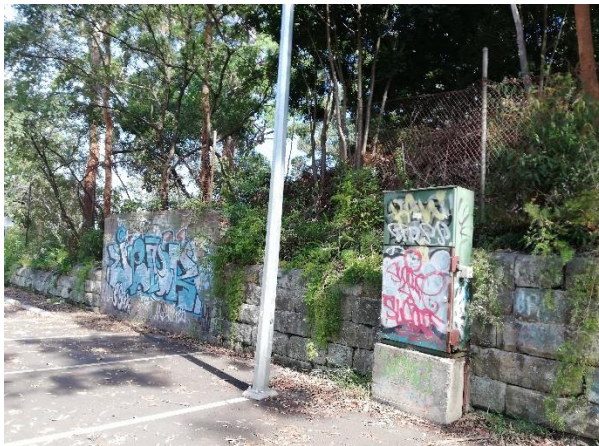
Figure 12: View along the retaining wall, note the graffiti on the brick portion and the different wall heights
