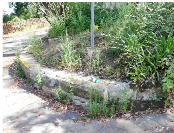
Figure 15: Sandstone curb adjacent to the southern side of the driveway using the same stone as the retaining wall
