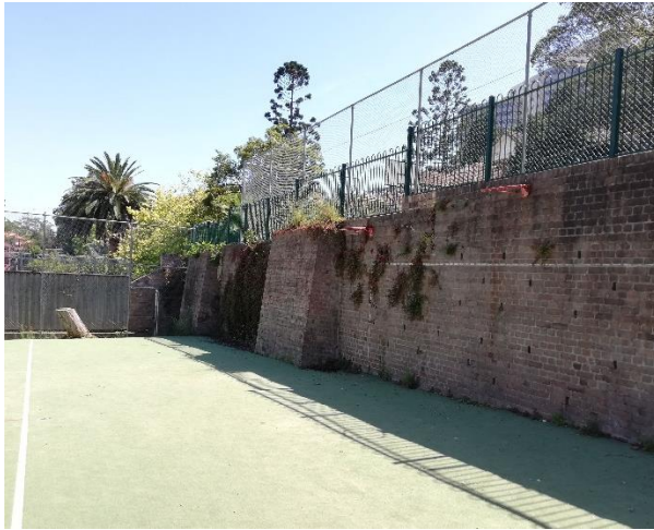
Figure 7: Brick retaining wall adjacent to the basketball court in the area known as the Loweres
