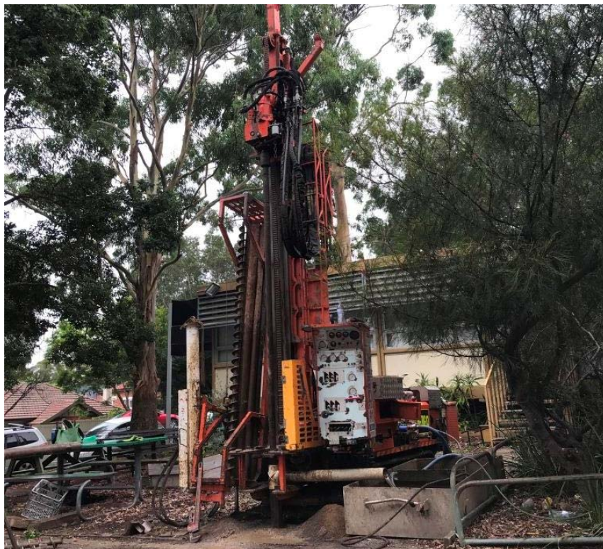
Photo 4: Typical Rig Coring setup - Centennial Avenue site facing East towards BH07
