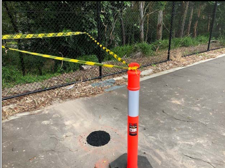
4. BH20 ISOLATED PATCHED HOLE WITH WARNING TAPE – 23.01.2019
