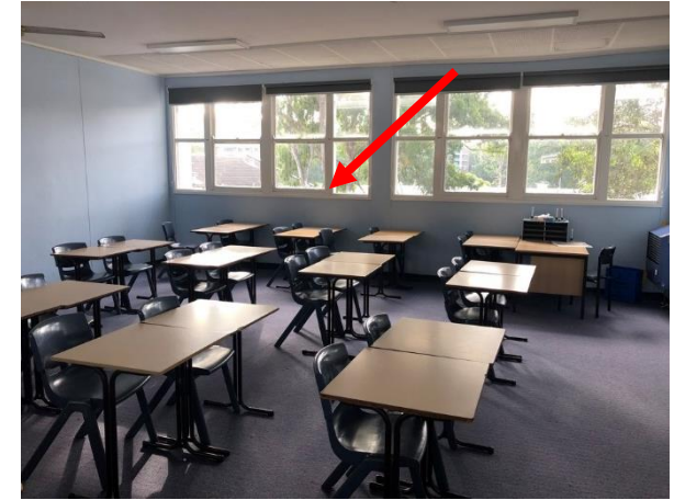
Photo 33: Building E, lead based white paint to Room R1007 windows
