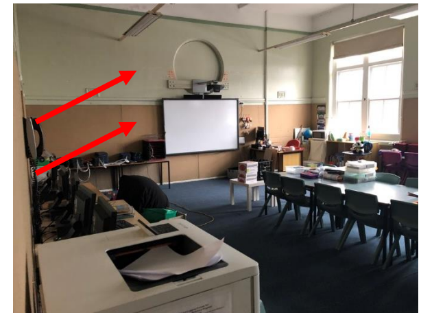
Photo 18: Building A, lead based green/orange paint to walls of Room R1012
