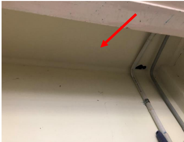
Photo 25: Building D, asbestos containing fibre cement sheeting to ceiling of Room R1012
