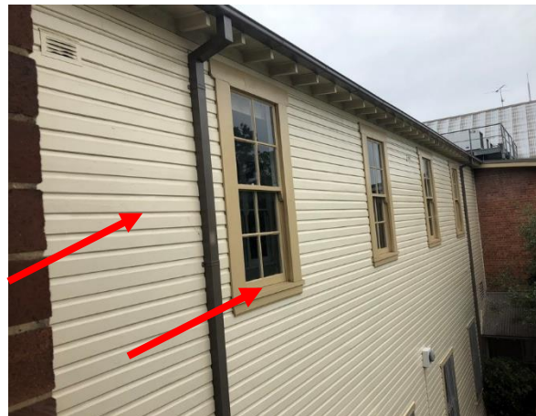
Photo 17: Building A, lead based cream paint to timber cladding and lead based tan paint to windows
