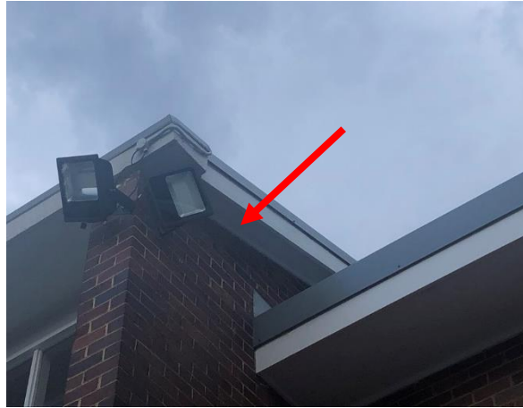
Photo 32: Building E, suspected asbestos containing fibre cement sheeting to eaves
