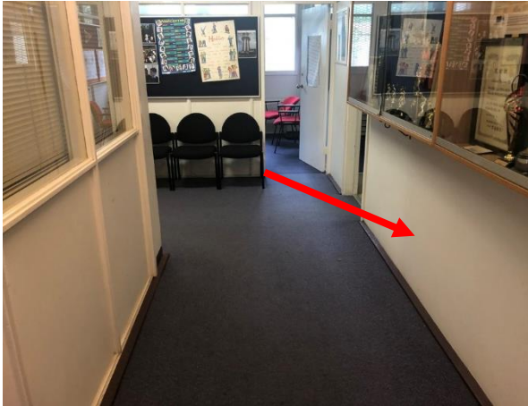
Photo 7: Building A, lead based cream paint to ground floor walls
