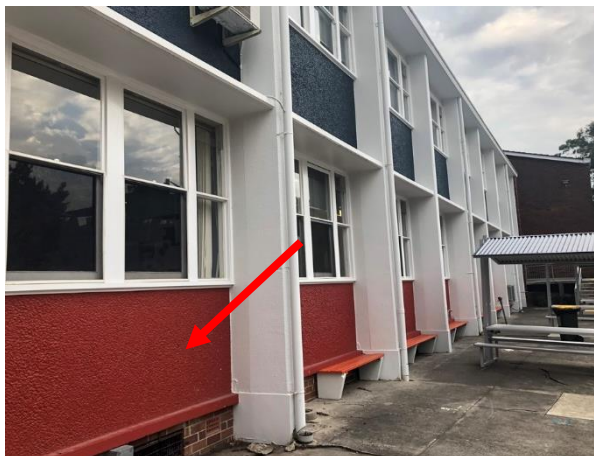
Photo 19: Building C, lead based orange/red paint to external walls
