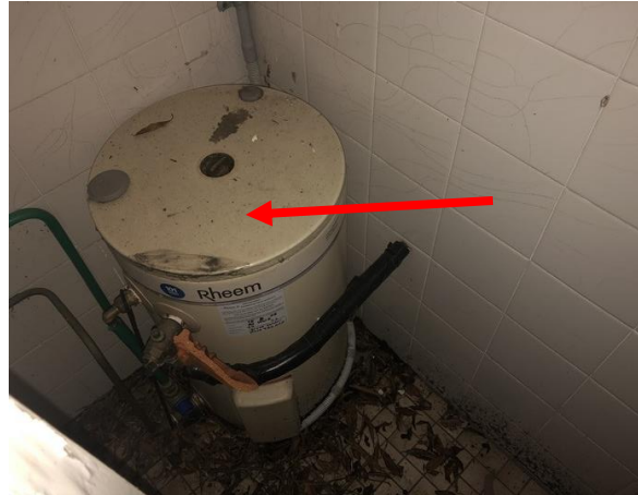
Photo 38: Building C, suspected SMF insulation core to hot water system in Room R0010
