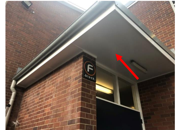
Photo 39: Building F, asbestos containing fibre cement sheeting to east and west entry soffits (R0017 & R0018)
