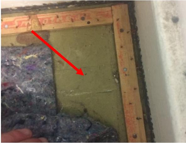
Photo 25: Building B, asbestos containing olive vinyl floor tiles to Room R1007
