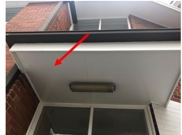
Photo 18: Building C, asbestos containing fibre cement sheeting to east and west entry soffits (R0013 & R0016)
