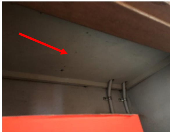
Photo 11: Building B, asbestos containing fibre cement sheeting to ceiling of Room R0008
