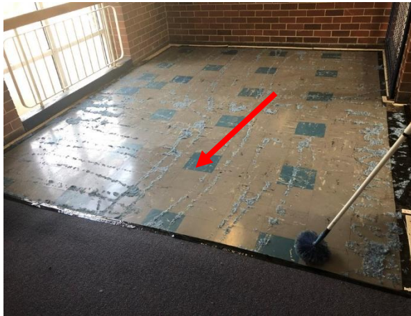
Photo 37: Building F, asbestos containing light blue vinyl floor tiles to Room R1012
