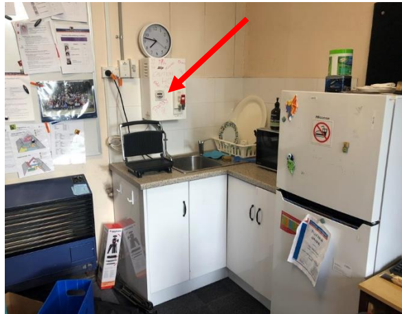
Photo 35: Building E, suspected SMF internal insulation core to instant hot water system in Room R0010
