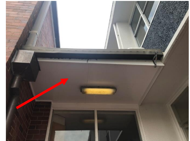
Photo 3: Building A, asbestos containing fibre cement sheeting to east and west entry soffits (R011 & R017)
