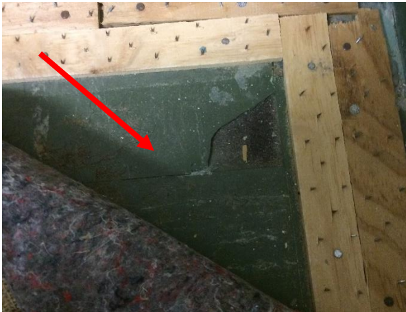
Photo 4: Building A, asbestos containing green vinyl floor tiles to Room R1003
