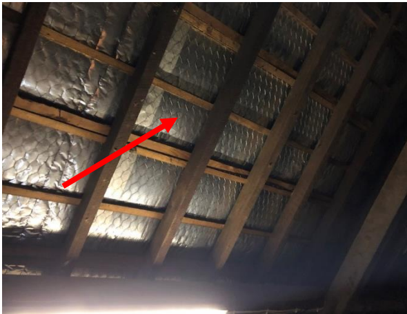
Photo 22: Building A, suspected SMF insulation to roof sarking
