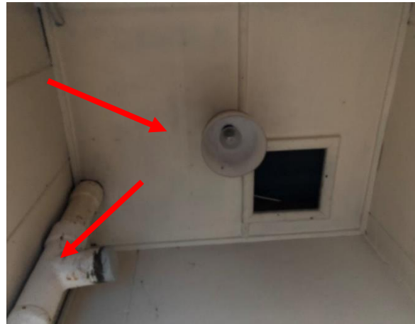
Photo 17: Building C, asbestos containing fibre cement sheeting to the ceiling and asbestos containing fibre cement flue pipe in Room R0017
