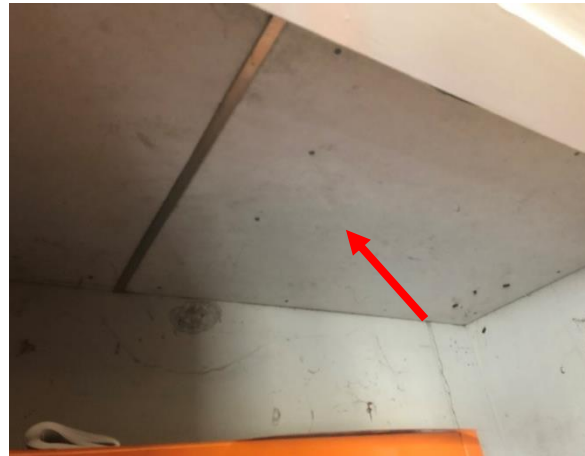
Photo 38: Building C, asbestos containing fibre cement sheeting to ceiling of Room R1004
