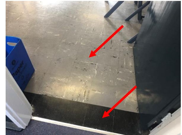
Photo 36: Building F, asbestos containing grey and black vinyl floor tiles to Room R1019
