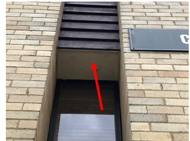
Photo 54: Building J, suspected asbestos containing fibre cement sheeting to eaves above windows
