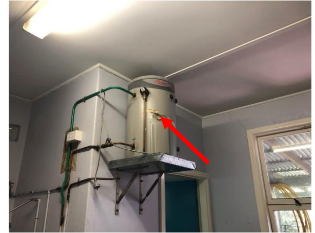
Photo 57: Building AA, suspected SMF insulation core to hot water system in Room R0007
