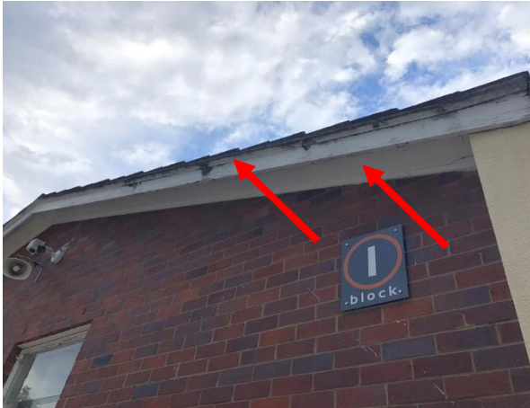
Photo 49: Building I, asbestos containing fibre cement sheeting to eaves and verge linings
