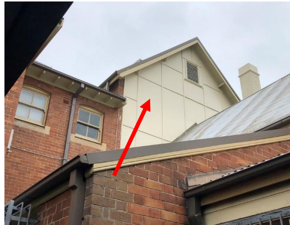
Photo 14: Building A, asbestos containing fibre cement sheeting to south gable
