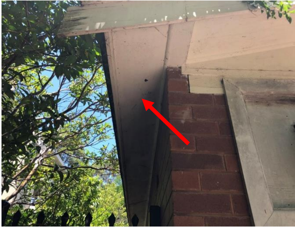
Photo 55: Building AA, asbestos containing fibre cement sheeting to eaves
