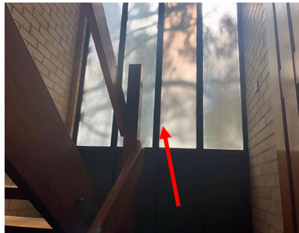
Photo 53: Building J, asbestos containing putty to aluminium framed windows
