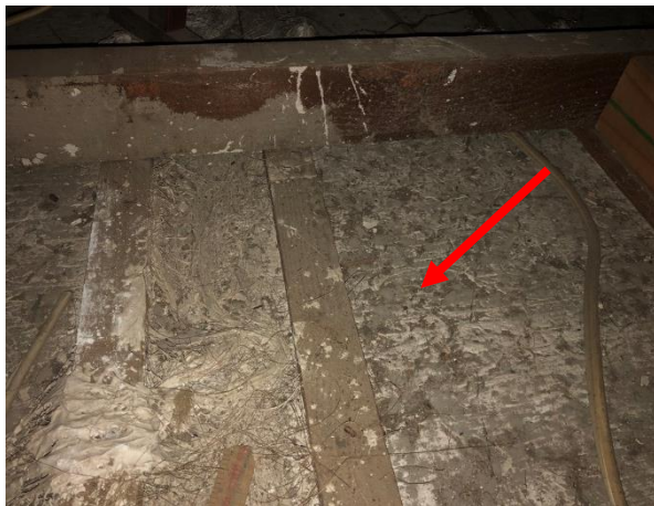
Photo 40: Building F, lead containing accumulated dust within roof void
