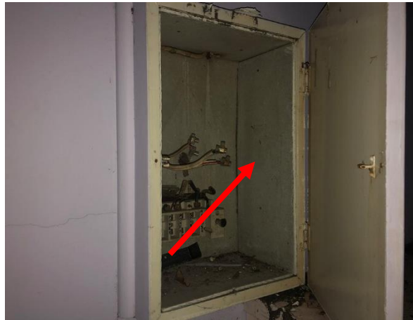
Photo 35: Building C, asbestos containing fibre cement sheeting to electrical panel in Room R0011
