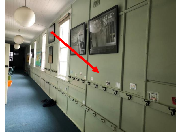
Photo 9: Building A, asbestos containing fibre cement sheeting to western wall of Room R1018
