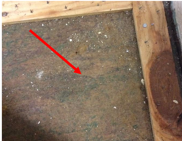
Photo 5: Building A, asbestos containing brown vinyl floor tiles to Room R1007
