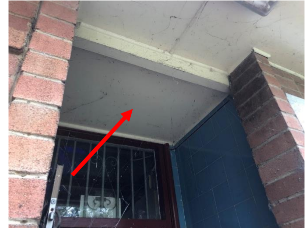
Photo 33: Building C, asbestos containing fibre cement sheeting to Room R0001 ceiling (external soffit)
