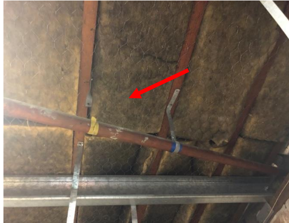
Photo 44: Building H, suspected SMF insulation to roof sarking
