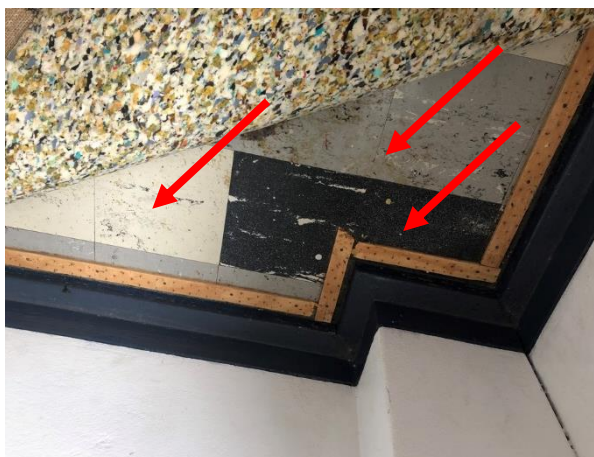
Photo 22: Building D, asbestos containing grey, black and cream vinyl floor tiles to Room R1001
