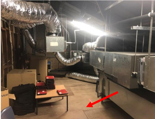
Photo 43: Building H, lead containing accumulated dust to the floor of Room M2008
