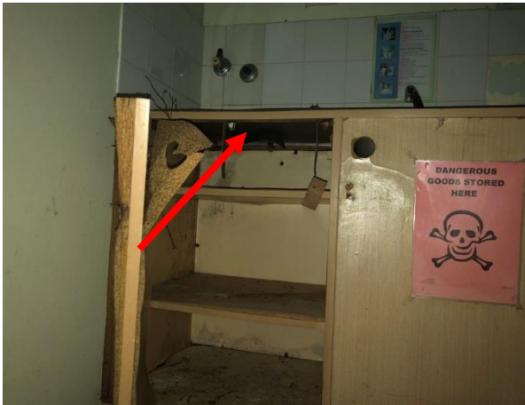
Photo 34: Building C, asbestos containing bituminous pad under sink in Room R0004
