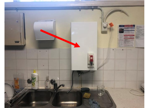
Photo 9: Building A, suspected SMF insulation core to instant hot water system in Room R0014
