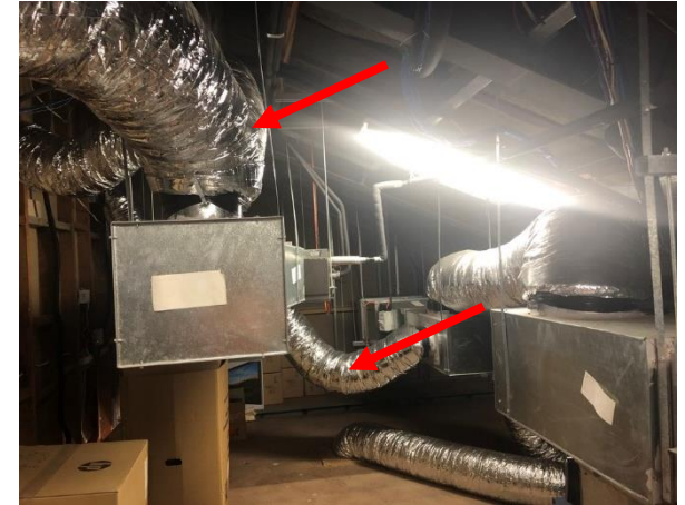
Photo 45: Building H, suspected SMF insulation to air conditioning ducting
