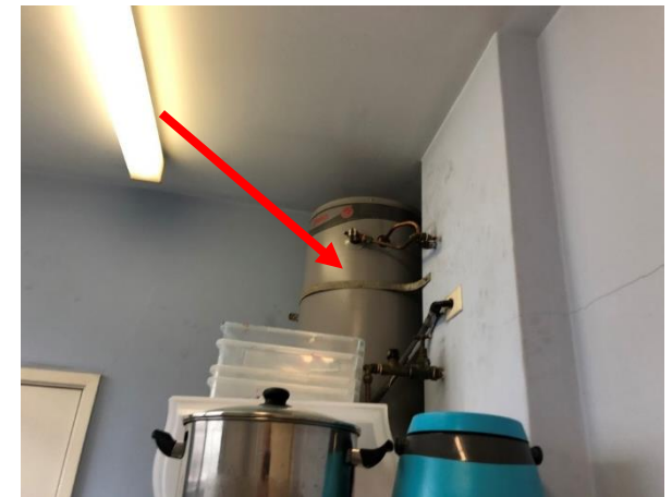
Photo 42: Building H, suspected SMF insulation core to hot water system in Room R0016
