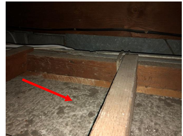
Photo 6: Building A, lead containing accumulated dust throughout roof void
