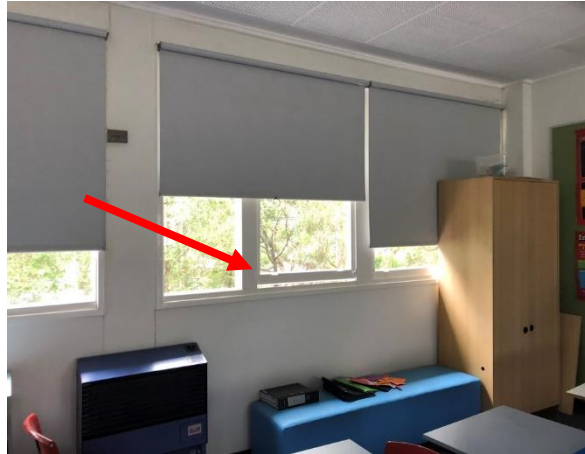
Photo 8: Building A, lead based white paint to Room R1001 windows
