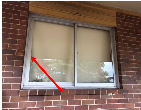
Photo 41: Building H, assumed asbestos containing putty to aluminium windows
