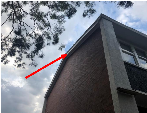
Photo 4: Building A, suspected asbestos containing fibre cement sheet eaves and verge linings
