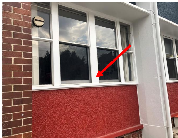
Photo 20: Building C, lead based white paint to external windows
