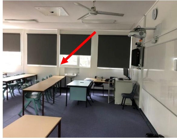
Photo 14: Building B, lead based cream paint to first floor internal windows
