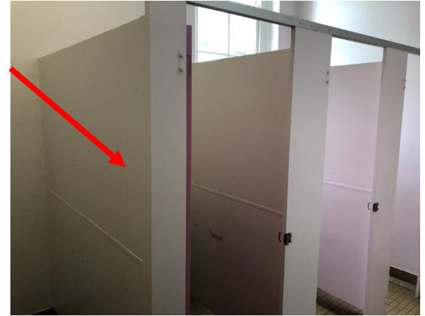
Photo 27: Building B, asbestos containing fibre cement cubicle partitions to Room R0004
