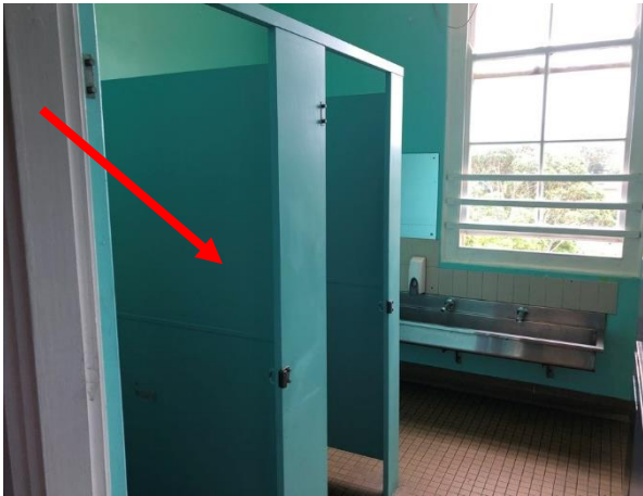
Photo 28: Building B, asbestos containing fibre cement cubicle partitions to Room R1003
