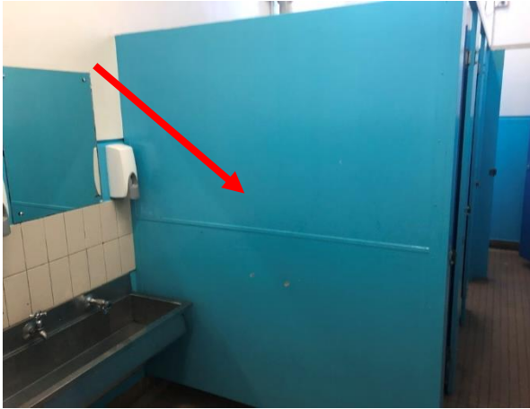
Photo 7: Building A, asbestos containing fibre cement cubicle partitions to Room R0023
