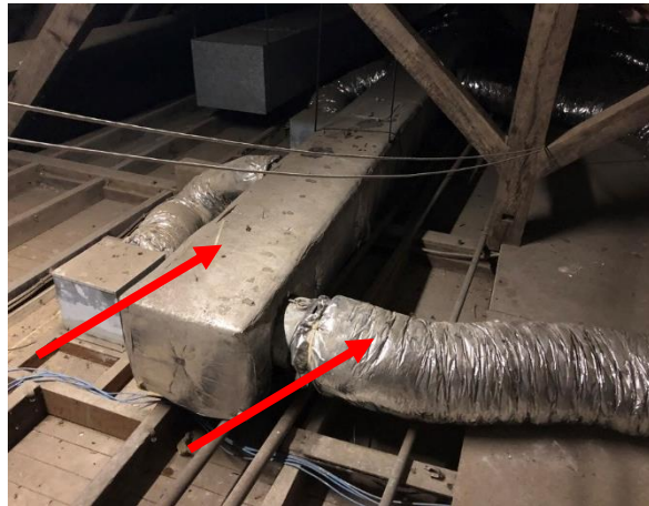
Photo 23: Building A, suspected SMF insulation lagging to air conditioning ducting
