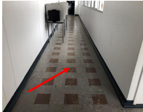
Photo 2: Building A, asbestos containing brown vinyl floor tiles to Room R1010
