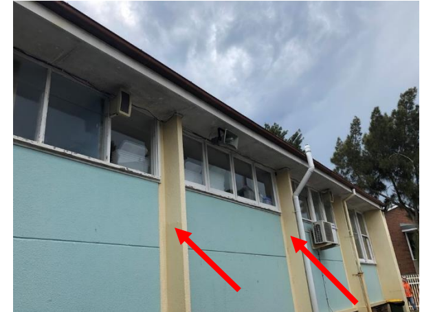
Photo 51: Building I, lead based cream paint to external walls
