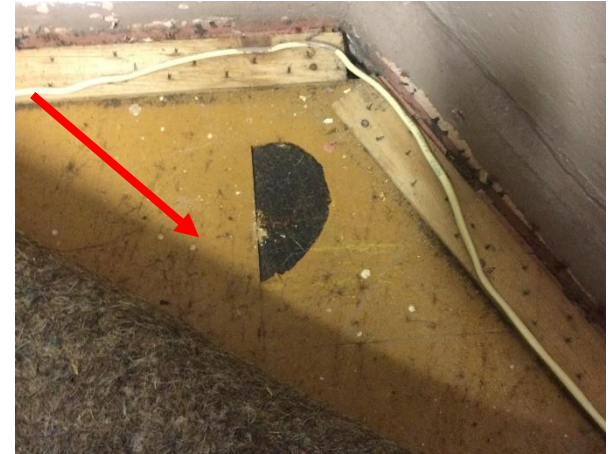
Photo 3: Building A, asbestos containing mustard vinyl floor tiles to Room R0031
