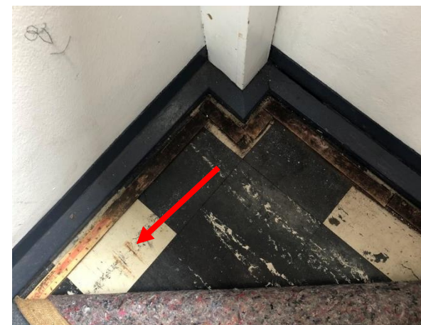
Photo 24: Building D, asbestos containing white vinyl floor tiles to Room R1010
