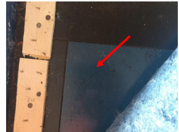
Photo 30: Building E, asbestos containing blue vinyl floor tiles to Room R1001
