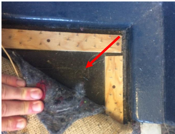
Photo 28: Building E, asbestos containing black vinyl floor tiles to Room R0007
