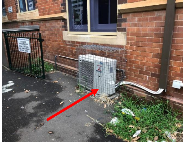
Photo 20: Building A, suspected internal SMF insulation to air conditioning units
