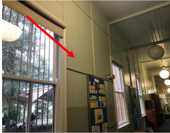
Photo 8: Building A, asbestos containing fibre cement sheeting to western wall of Room R0031
