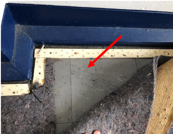
Photo 16: Building C, asbestos containing grey vinyl floor tiles to Room R1008
