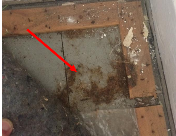
Photo 26: Building B, asbestos containing grey vinyl floor tiles to Room R1015
