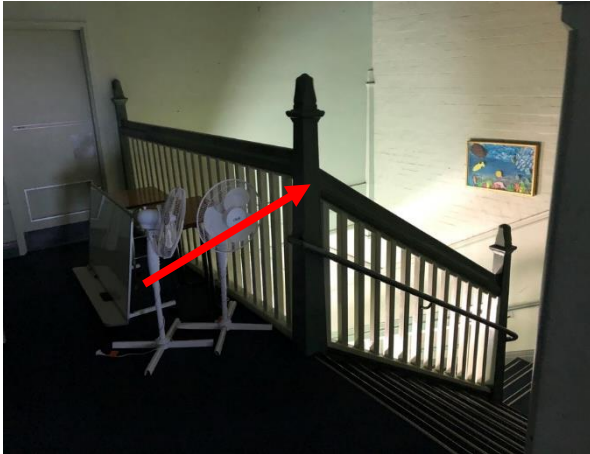
Photo 19: Building A, lead based green paint to stair handrail in Room R1020
