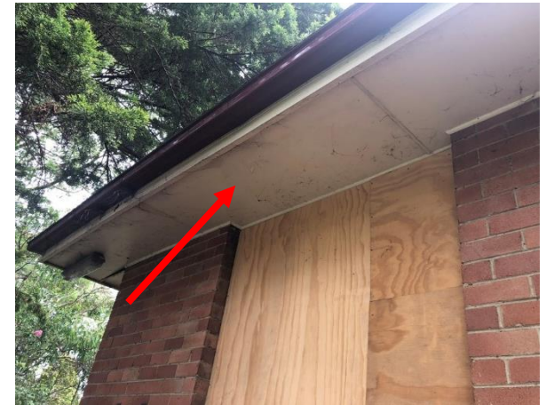
Photo 36: Building C, asbestos containing fibre cement eaves
