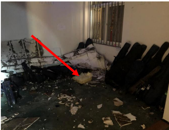
Photo 40: Building C, suspected SMF insulation debris throughout internal areas
