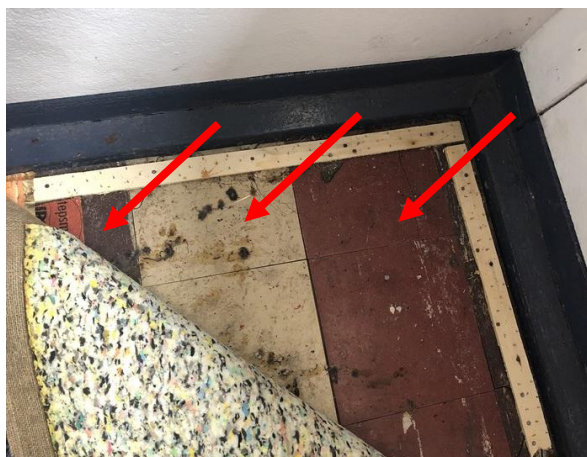
Photo 23: Building D, asbestos containing red, beige and brown vinyl floor tiles to Room R1002
