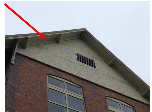
Photo 12: Building A, suspected asbestos containing fibre cement eaves
