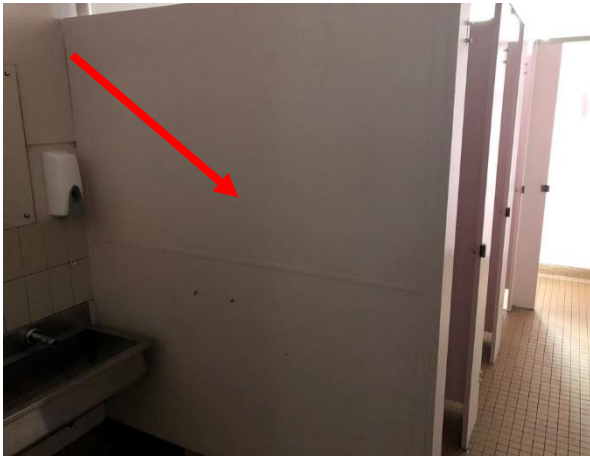
Photo 10: Building A, asbestos containing fibre cement cubicle partitions to Room R1005
