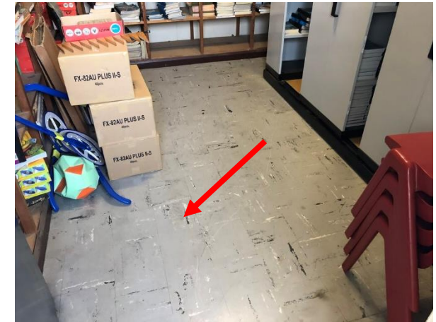
Photo 27: Building E, asbestos containing grey vinyl floor tiles to Room R1004
