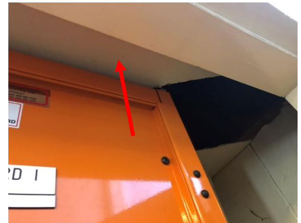
Photo 48: Building I, asbestos containing fibre cement sheet ceiling to Room R0007
