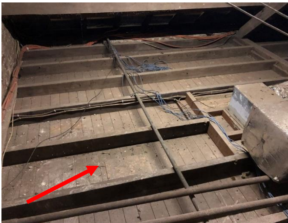
Photo 16: Building A, lead containing dust within roof void
