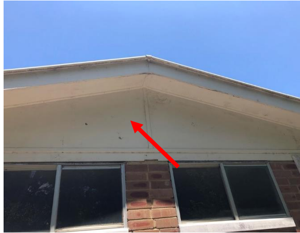
Photo 56: Building AA, asbestos containing fibre cement sheeting to gable panels
