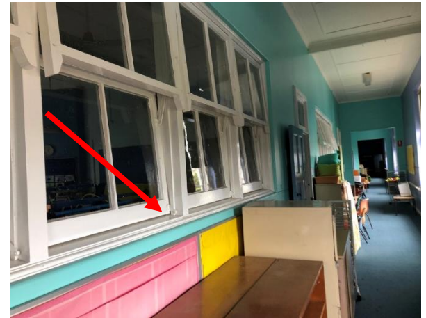
Photo 30: Building B, lead based white paint to windows in Room R1005
