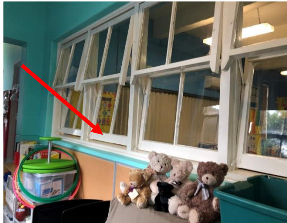
Photo 29: Building B, lead based white paint to windows in Room R0008
