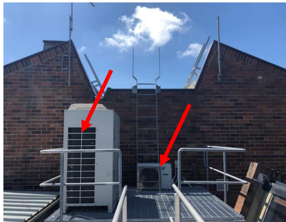
Photo 47: Building H, suspected SMF internal insulation to air conditioning units
