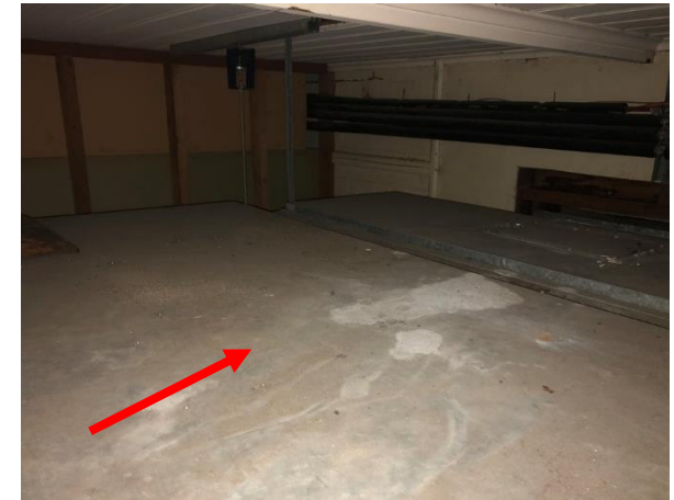
Photo 15: Building A, lead containing dust to air conditioning loft in Room R0031
