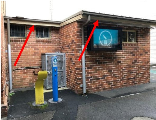
Photo 13: Building A, asbestos containing fibre cement eaves to R0022 and R0044
