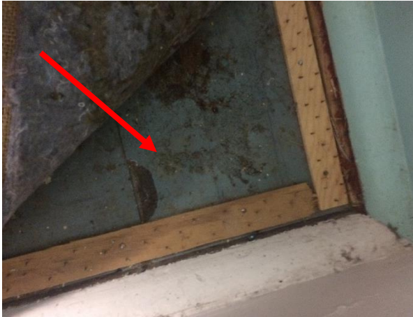
Photo 1: Building A, asbestos containing green vinyl floor tiles to Room R0001
