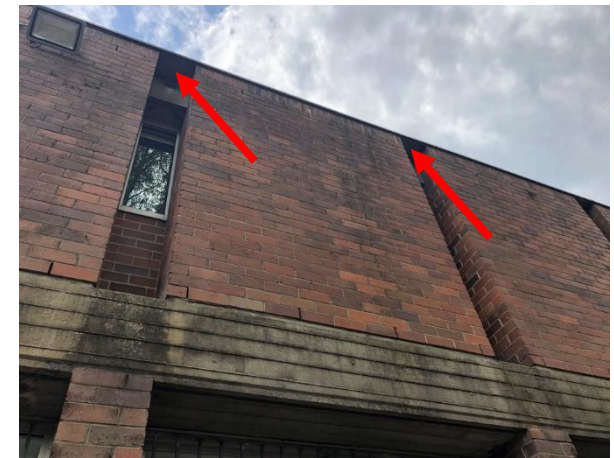
Photo 42: Building H, suspected asbestos containing fibre cement sheeting to eaves above windows
