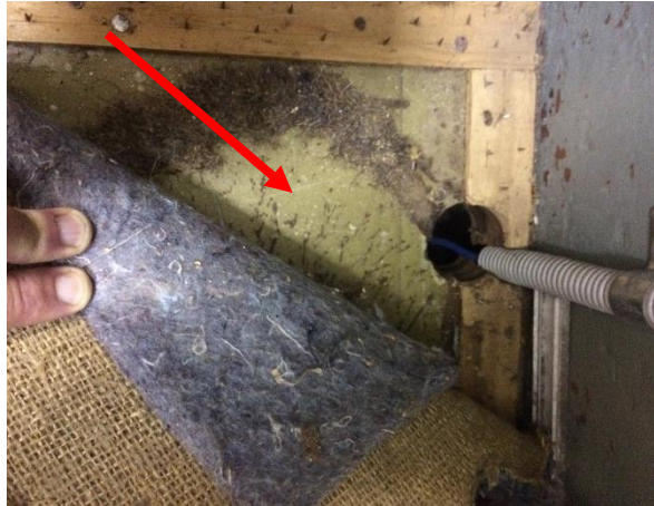
Photo 2: Building A, asbestos containing beige vinyl floor tiles to Room R0010
