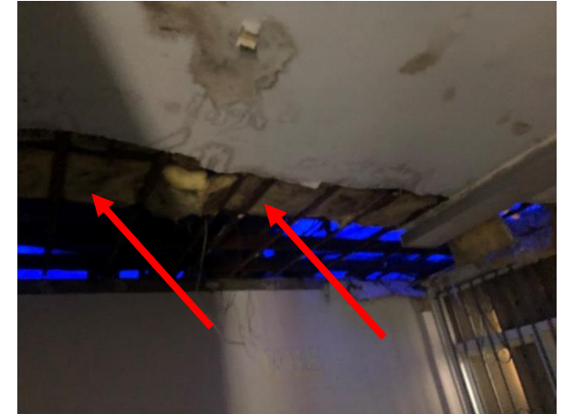
Photo 39: Building C, suspected SMF insulation throughout roof void
