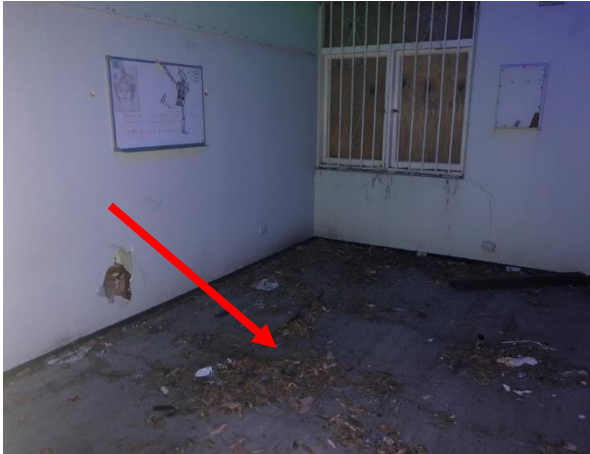
Photo 37: Building C, lead containing dust to Room R0015
