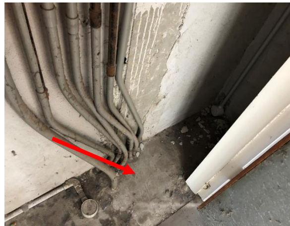
Photo 5: Building A, asbestos containing accumulated dust to floor of Room R1007
