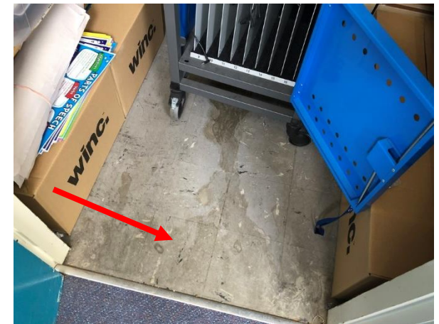
Photo 12: Building B, asbestos containing grey vinyl floor tiles to Room R1004
