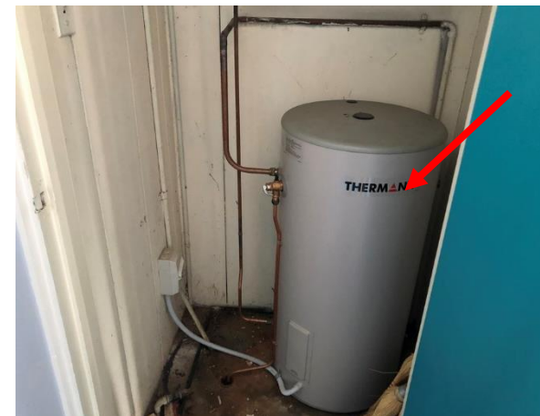
Photo 21: Building C, suspected SMF insulation core to hot water system in Room R0017
