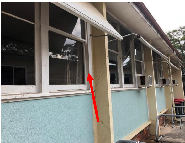
Photo 52: Building I, lead based white paint to external windows
