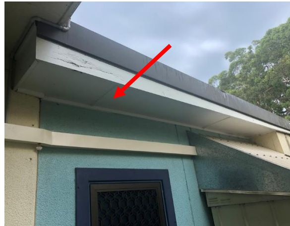
Photo 26: Building D, asbestos containing fibre cement sheeting to the external eaves of Room R0026
