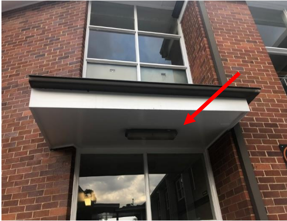
Photo 31: Building E, asbestos containing fibre cement sheeting to east and west entry soffits (R0014, R0020 & R0021)
