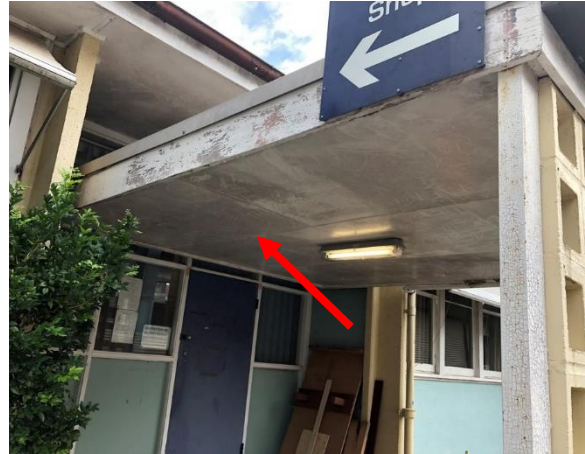
Photo 50: Building I, asbestos containing fibre cement sheeting to external soffit lining (R0017)
