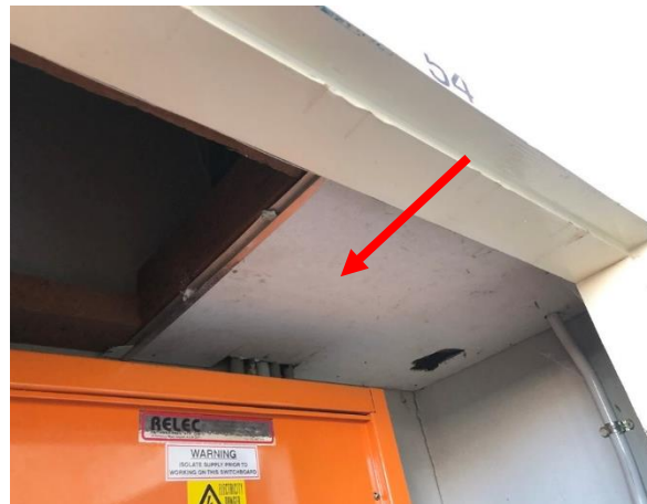
Photo 29: Building E, asbestos containing fibre cement sheeting to ceiling of Room R0009
