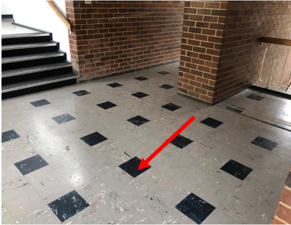
Photo 13: Building B, asbestos containing blue vinyl floor tiles to Room R1010
