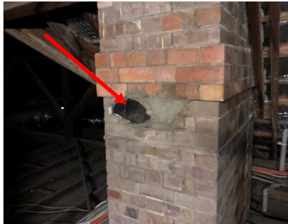
Photo 11: Building A, asbestos containing fibre cement chimney flue pipe in roof void
