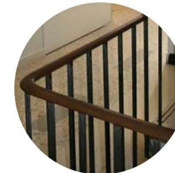
HR2 - HANDRAIL TYPE 3 BRONZE HANDRAIL (TO MATCH EXISTING) LOCATION: RELOCATED FIRE STAIR DESIGN INTENT: ECHO OF THE ORIGINAL STAIR
