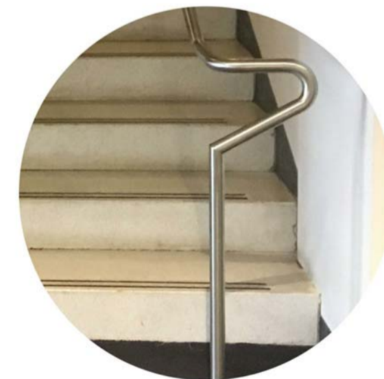
STAINLESS STEEL HANDRAIL LOCATION: ALL EXTERNAL HANDRAILS
