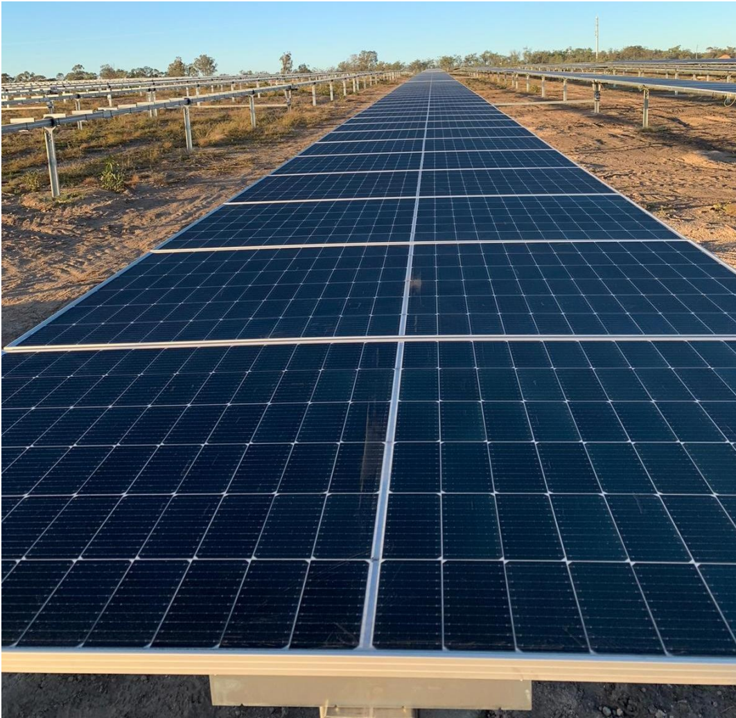
Figure 4-2 Typical single-axis tracking system
