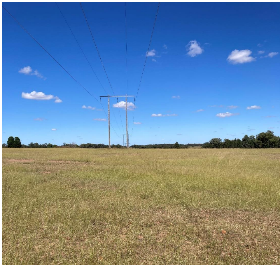
Figure 4-5 Existing 132kV transmission lines traversing the proposal site that will connect the solar farm to the Dubbo substation
