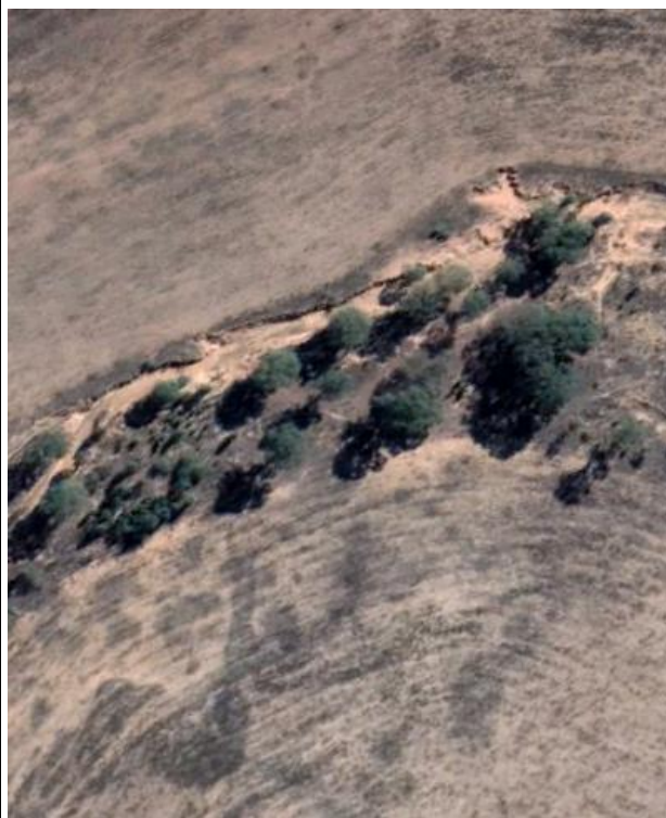
Figure 8-5 2019 Google Earth Aerial of bank erosion in creek
