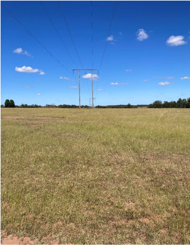
Figure 1-5 Existing transmission lines on site (preferred connection point)
