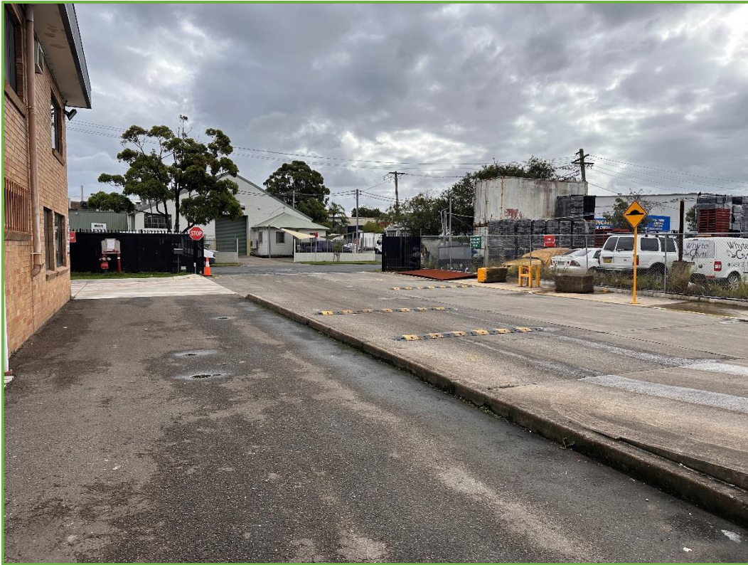
View looking west towards northern vehicular access
