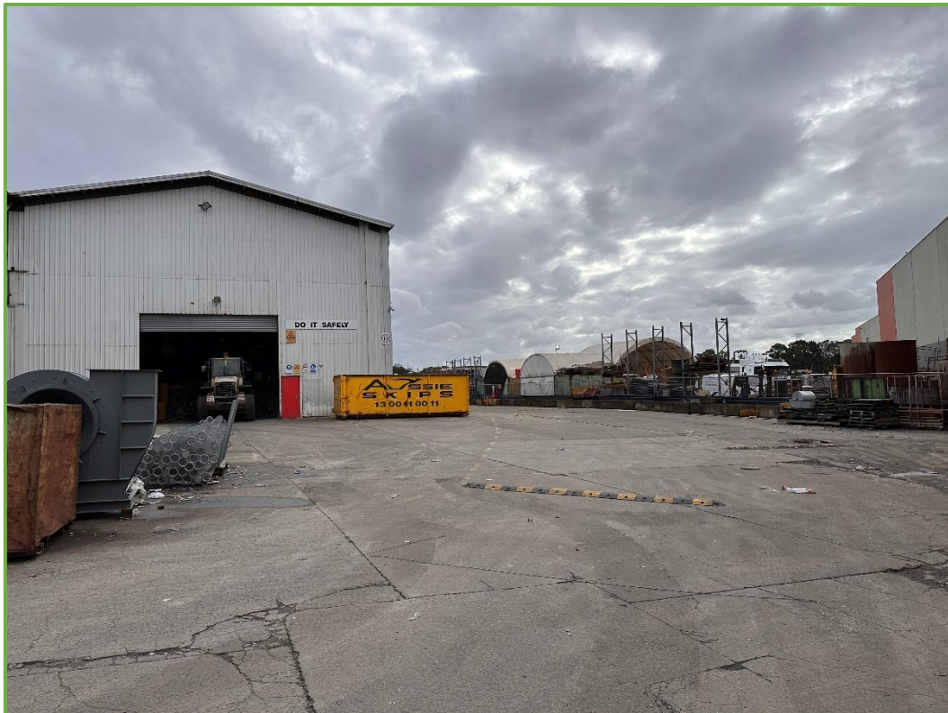
View looking west at end of northern internal roadway – towards glass processing area
