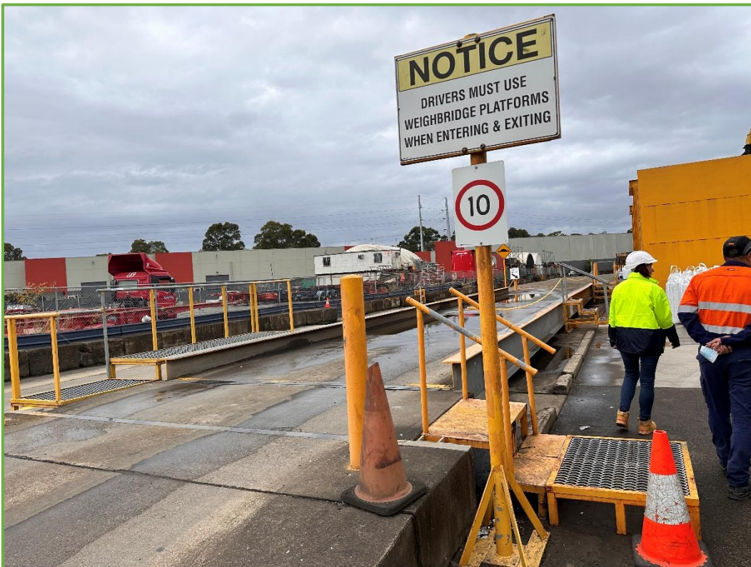
View looking east towards northern weighbridge
