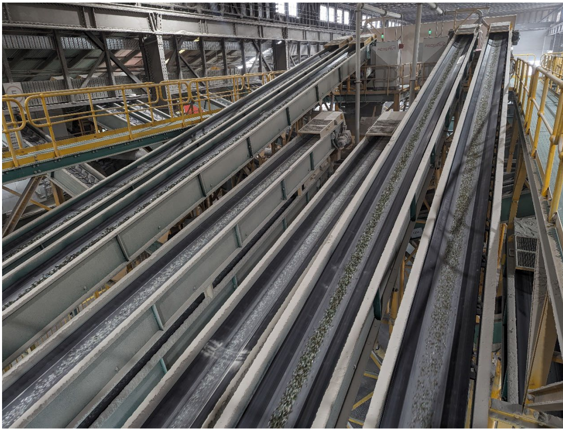
Figure 3-5: Conveyors transporting glass cullet to bunkers
