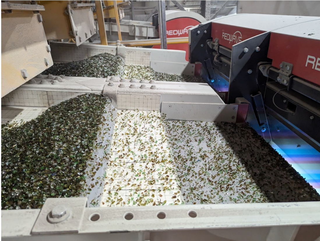
Figure 3-4: Optical Sorting Equipment
