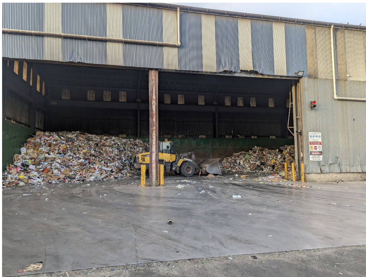
Figure 3-3: MRF Receiving Area
