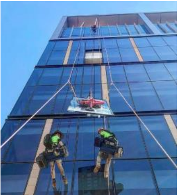
Glass Panel replacement
