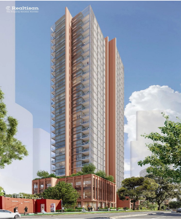
THE BRYSON 871-877 Pacific Highway
