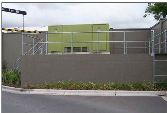
Figure 51 - Example substation raised above 1:100 flood level
