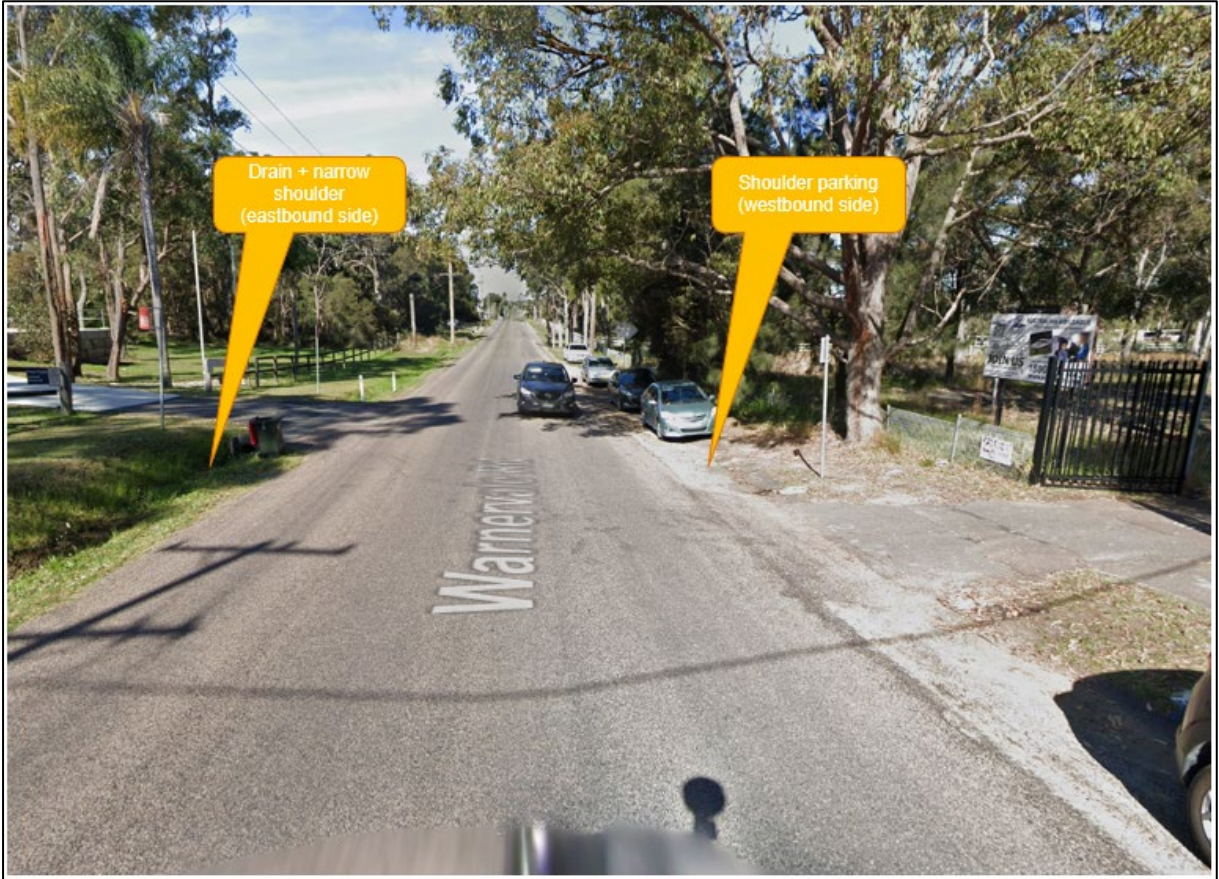
Figure 4: Warnervale Road frontage
