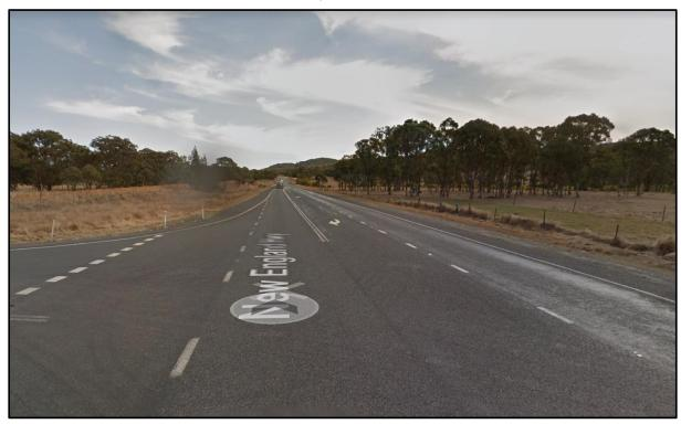
Photo 2 – Sheltered turn lane for right turning vehicles into Sunnyside Platform Road from the New England Highway. Note straight alignment that allow for good visibility
