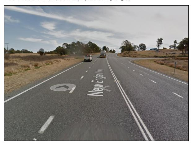
Photo 4 – View northbound on the New England Highway on approach to intersection with the Bruxner Highway. Note good forward visibility and dual lanes to allow a through vehicle movement to pass a left turning vehicle into the Bruxner Highway.
