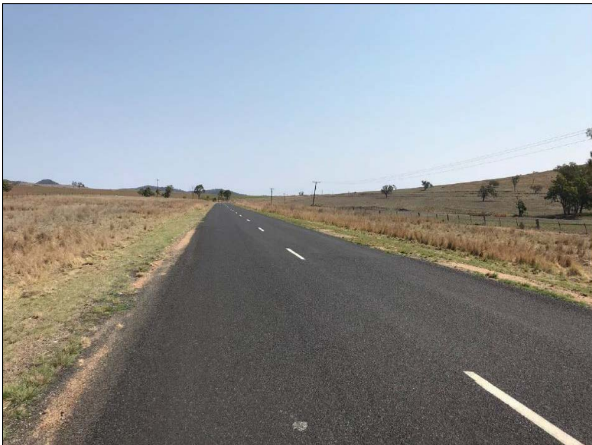
Figure 6-15 View along Bruxner Highway
