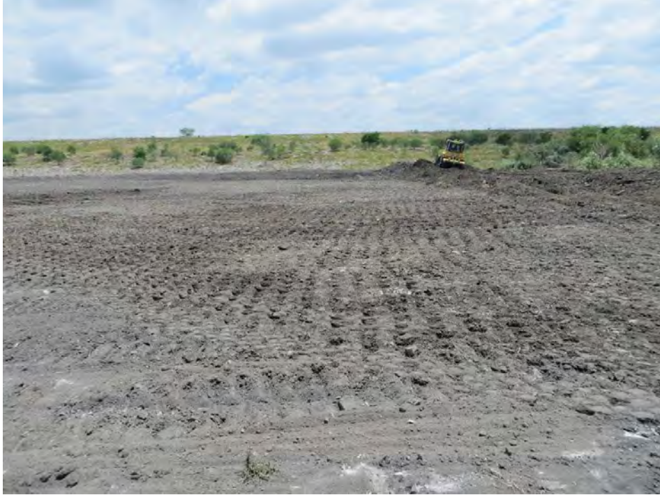
Photo 1 Looking north from the southern fringe over the prepared floor area
