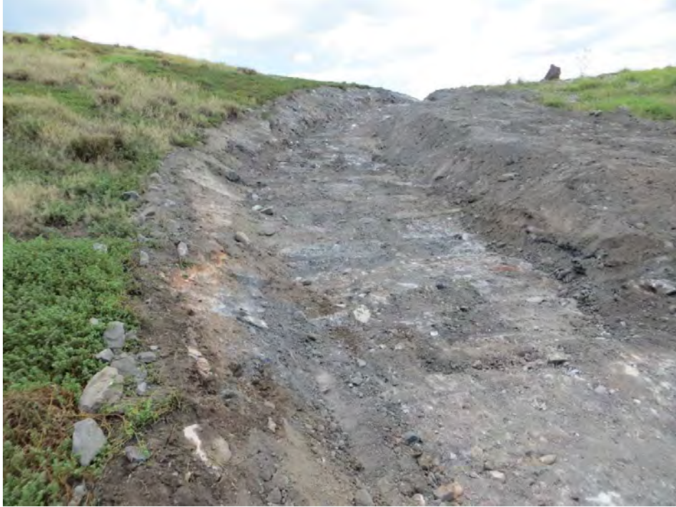
Photo 5 Channel connecting the composting pad and the sedimentation dam
