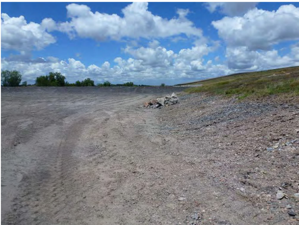
Photo 4 Looking south along the western fringe of the sedimentation basin
