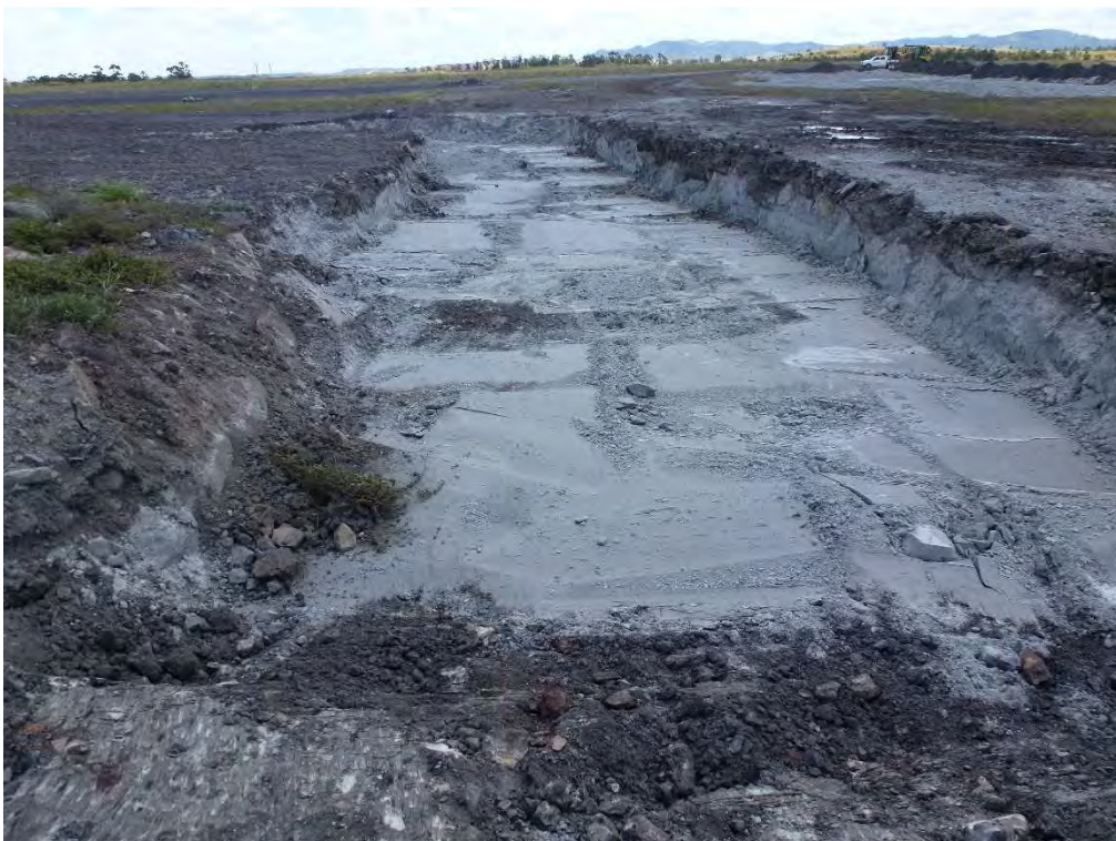
Photo 6 Approach of the overflow spillway channel
