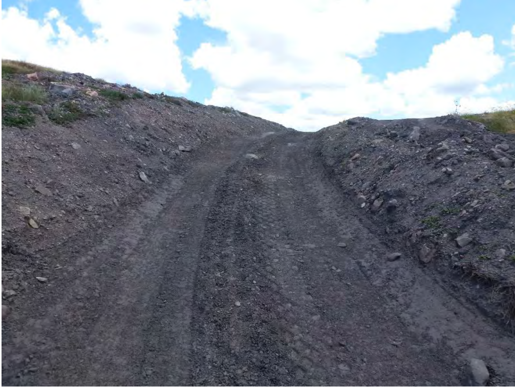
Photo 5 Channel connecting the composting pad and the sedimentation basin
