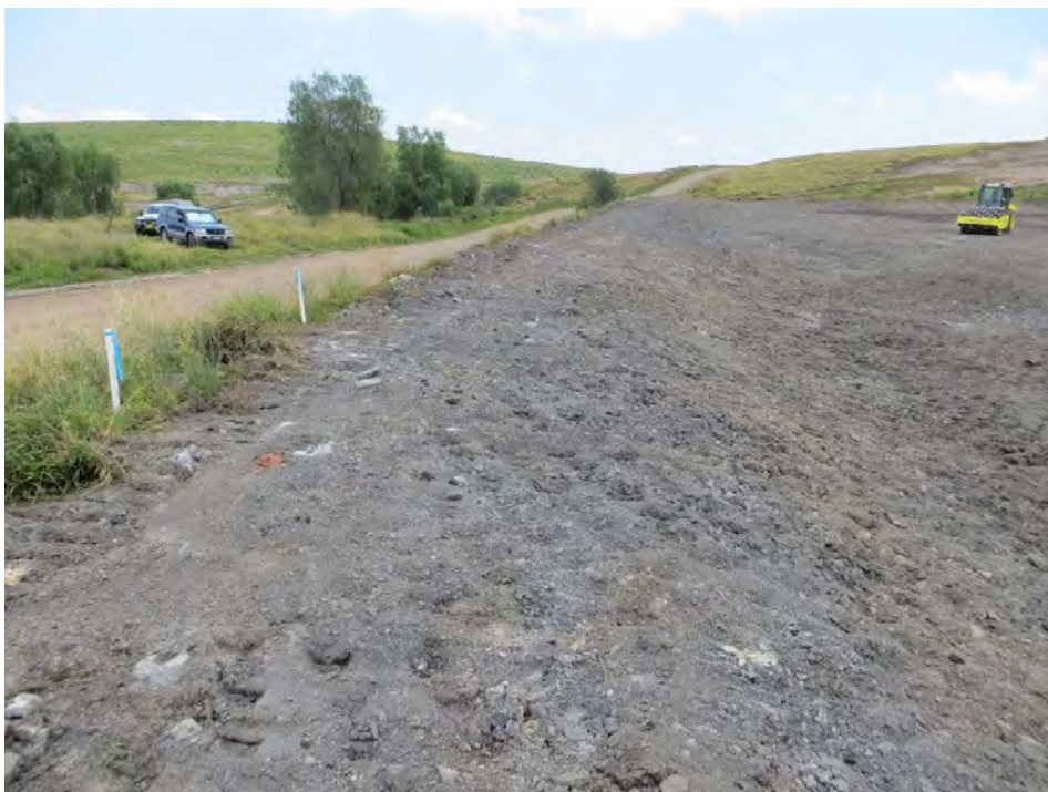
Photo 4 Looking west along the southern embankment
