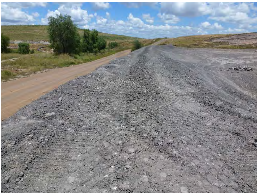
Photo 2 Looking west along the crest of the southern sedimentation basin embankment
