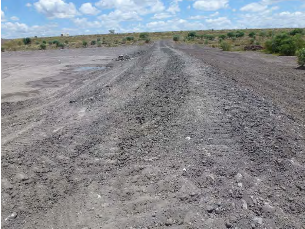
Photo 1 Looking north along the crest of the eastern sedimentation basin embankment
