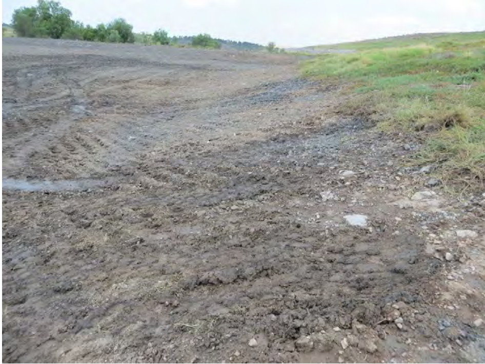
Photo 3 Looking south along the western perimeter prepared floor
