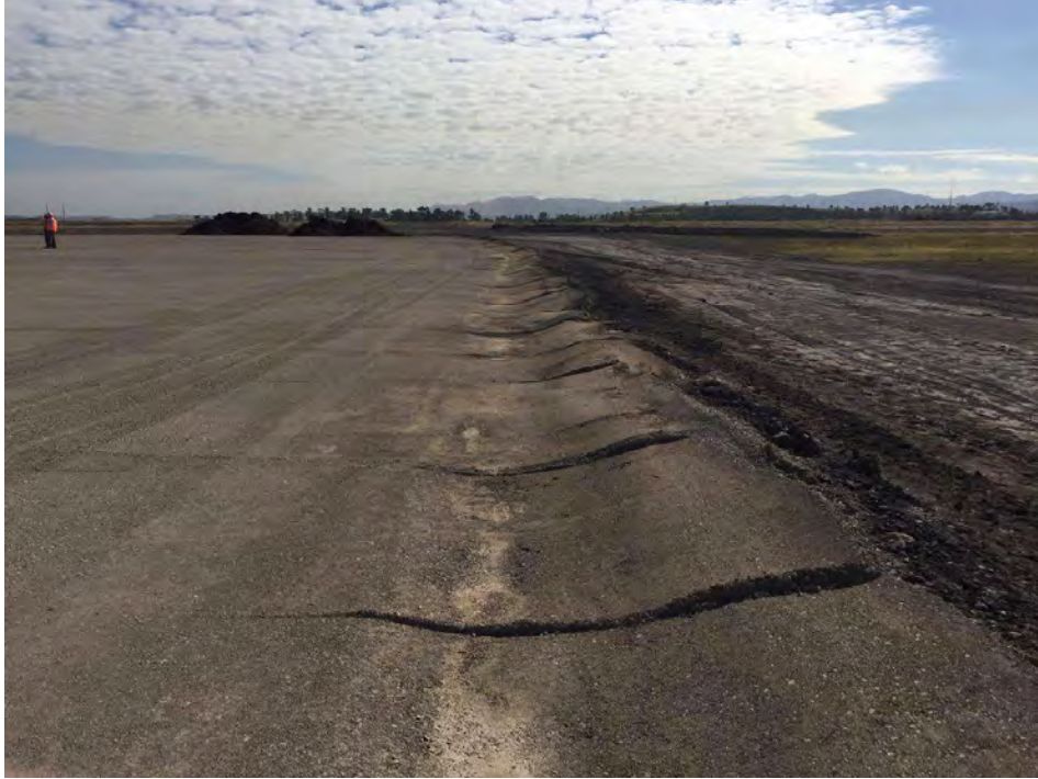
Photo 5 Looking along the composting pad eastern perimeter surface drain
