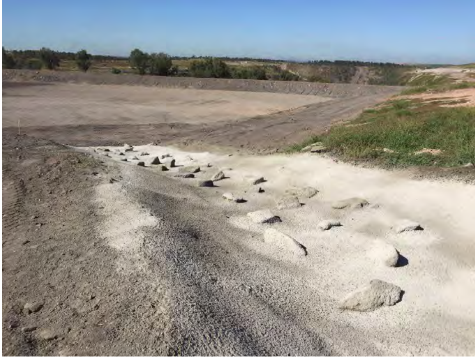
Photo 3 Looking down the shotcreted spillway channel
