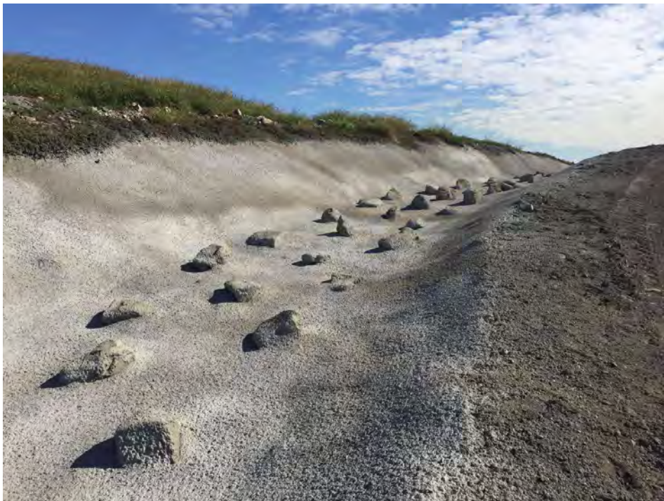
Photo 4 Looking up the shotcreted spillway channel
