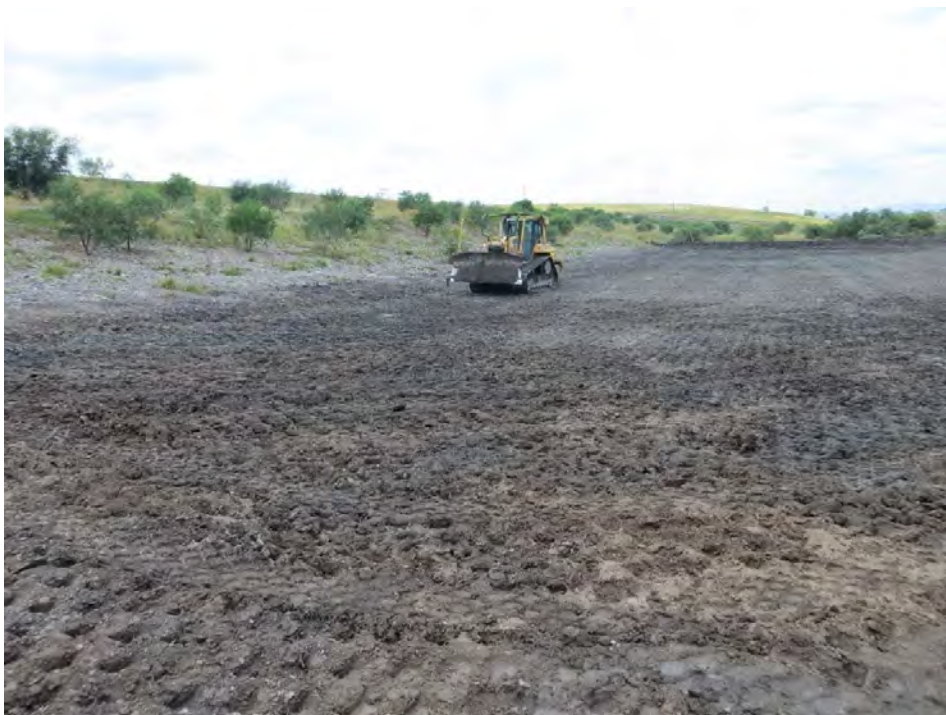
Photo 2 Looking east from the western fringe over the prepared floor area
