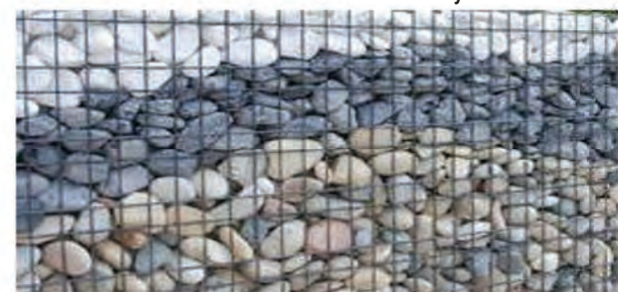
11 Gabion Feature Wall Finish or Similar
