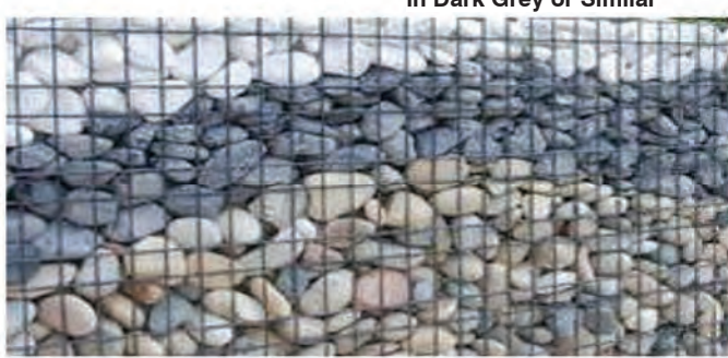
11 Gabion Feature Wall Finish or Similar
