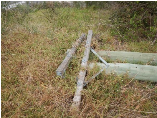
Figure 6.5: Fallen telephone pole (Photographed by R. Taddeucci, 24 September 2018)
