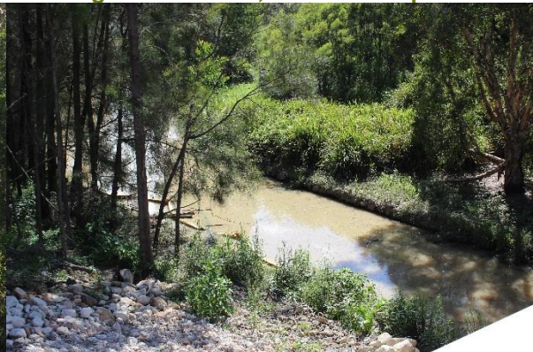
Figure 3.2: Boundary Creek with artificial retaining embankment, northeast aspect
