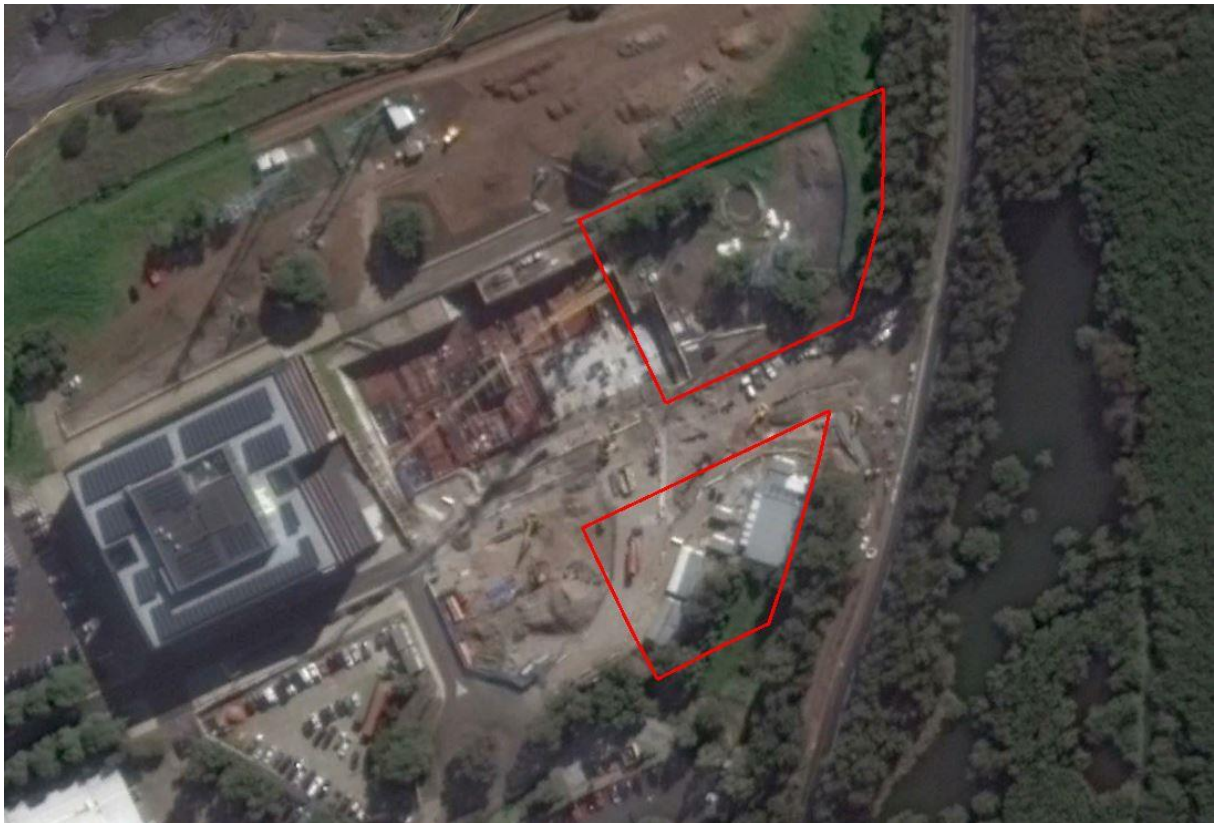
Figure 3.7: View of the study area in 2014 (Source: Google Earth)
