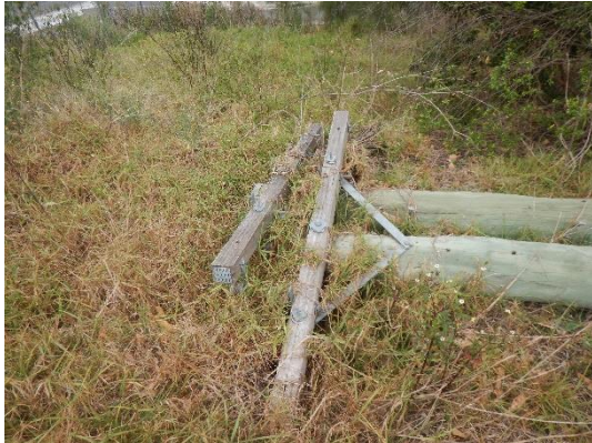
Figure 3.5: Fallen telephone pole (Photographed by R. Taddeucci, 24 September 2018)
