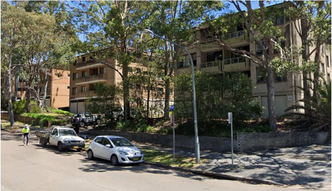
Figure 7 View looking west toward the subject buildings.
