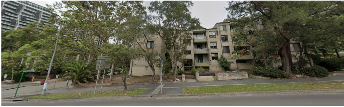
Photo 3 - Looking South-West Towards 21 Cottonwood Crescent from Waterloo Road (© Google Maps)
