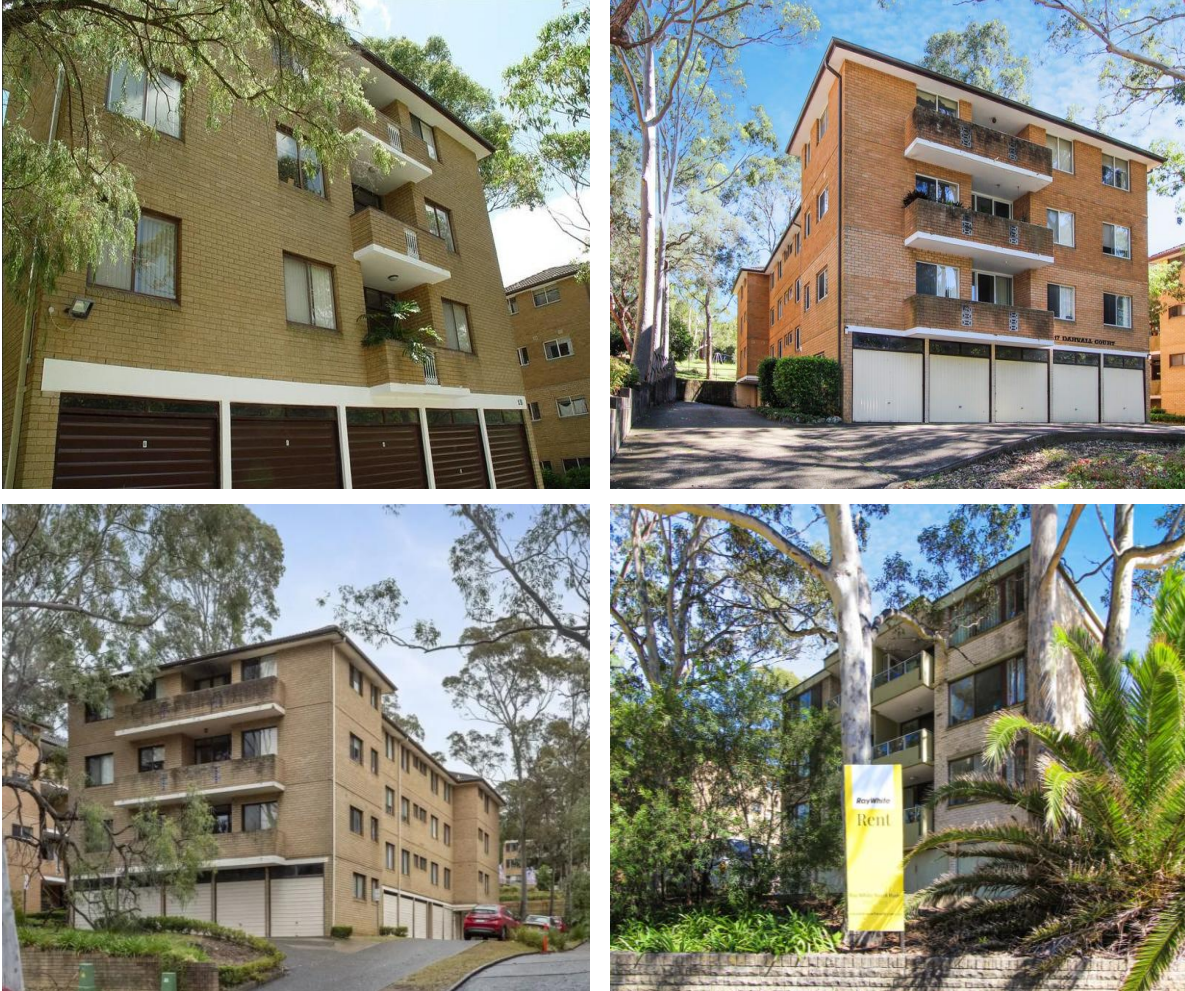
FIGURE 4-2: Existing Improvements, The Site
