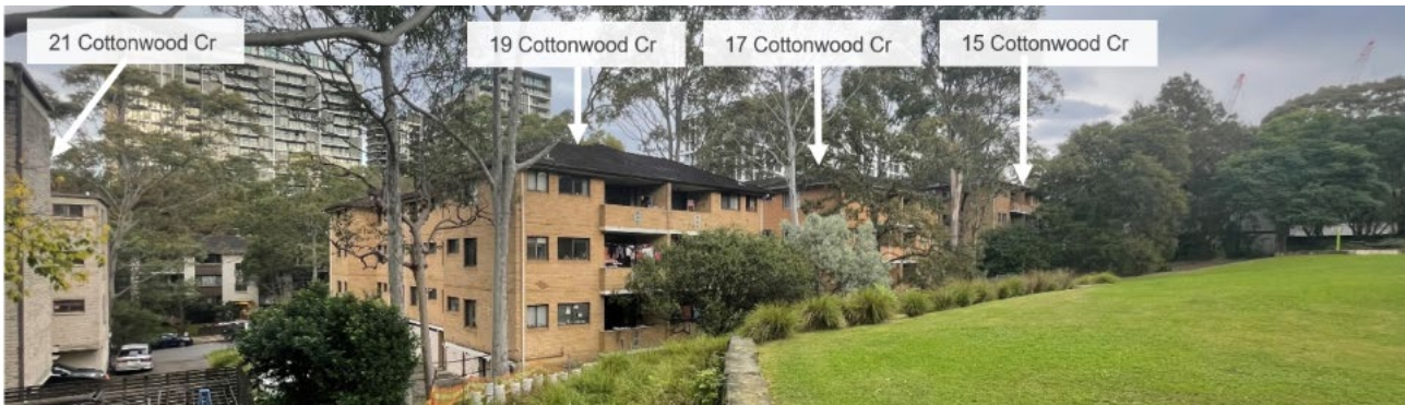
15-19 Cottonwood Cr: Facing east towards site from Elouera Reserve.
