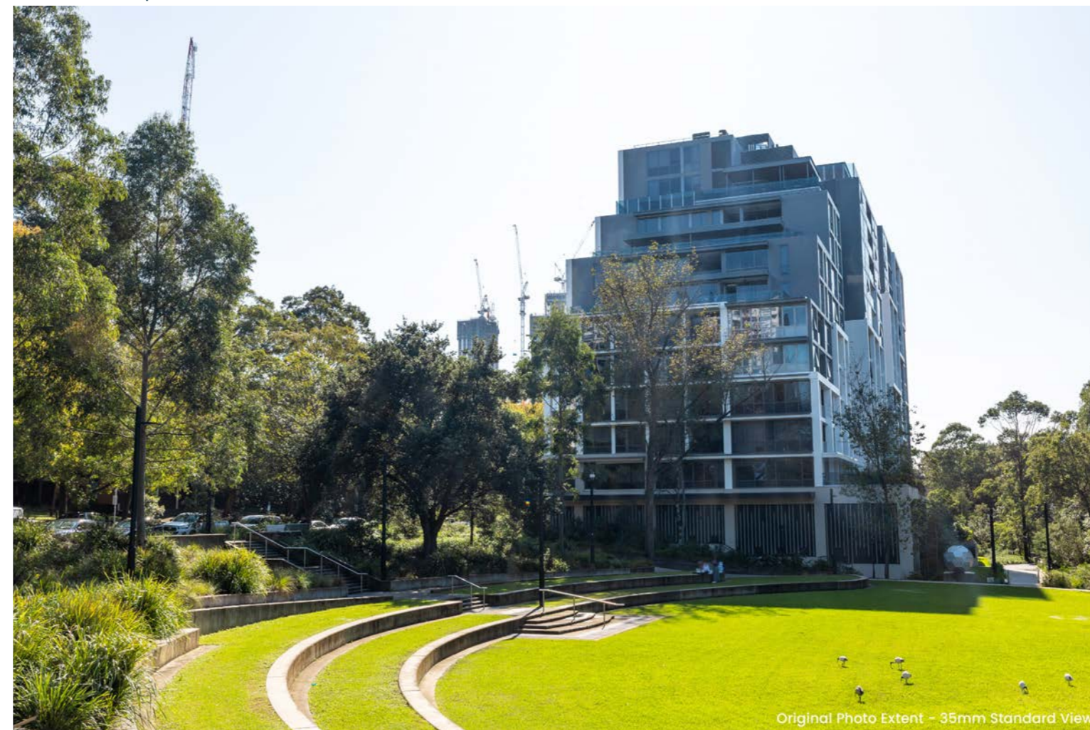
Figure 27 Viewpoint 03 existing view.
